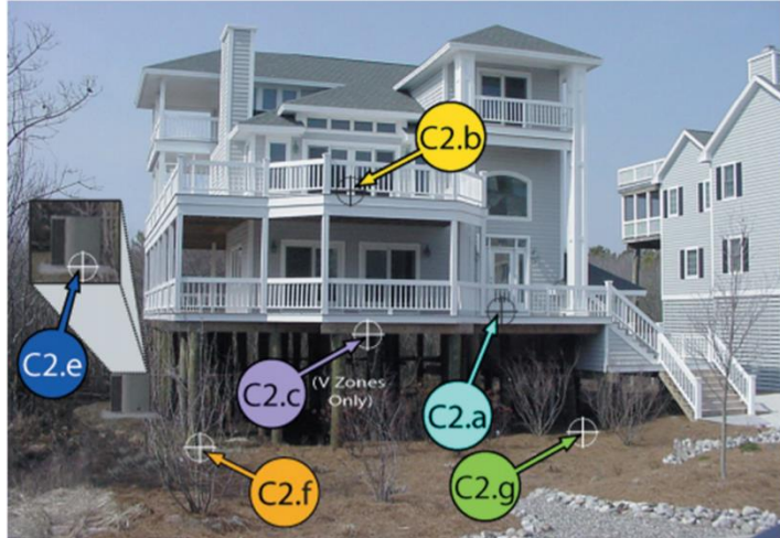
Figure 1: EC information collected shown on a housing unit (FEMA, 2020).
