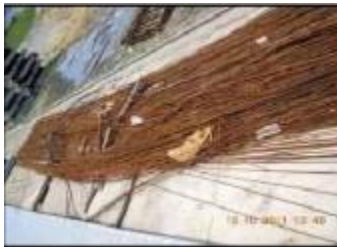
Surplus of reinforcement bar component waste
