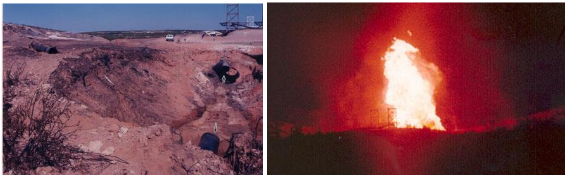
Figure 2 Crater formation and fire after pipeline rupture, New Mexico, USA Reprinted from [4]
