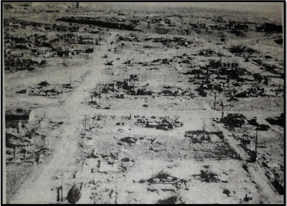
Figure10: Image of tornado damage. 21 The image highlighted the extreme damage and the document it was printed in “You and your city” push the unity narrative.
