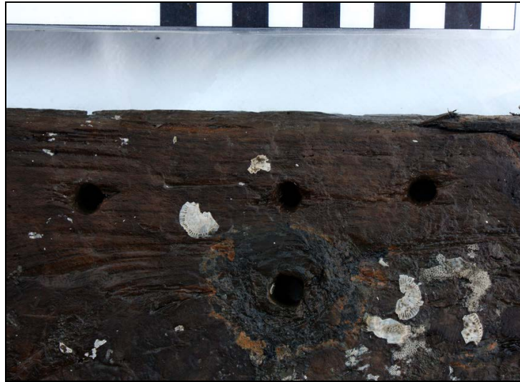
Figure A.2. Evidence for the use of a claw for the extraction of nails. Note sharp tool marks to either side of three disused nail holes, near edge; SS 7-6 (UM 31), outer face.
