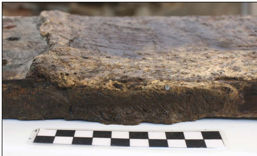
Figure 4.89. Caulk on lower edge of SS 3-5 at FR 22-FR 23.
