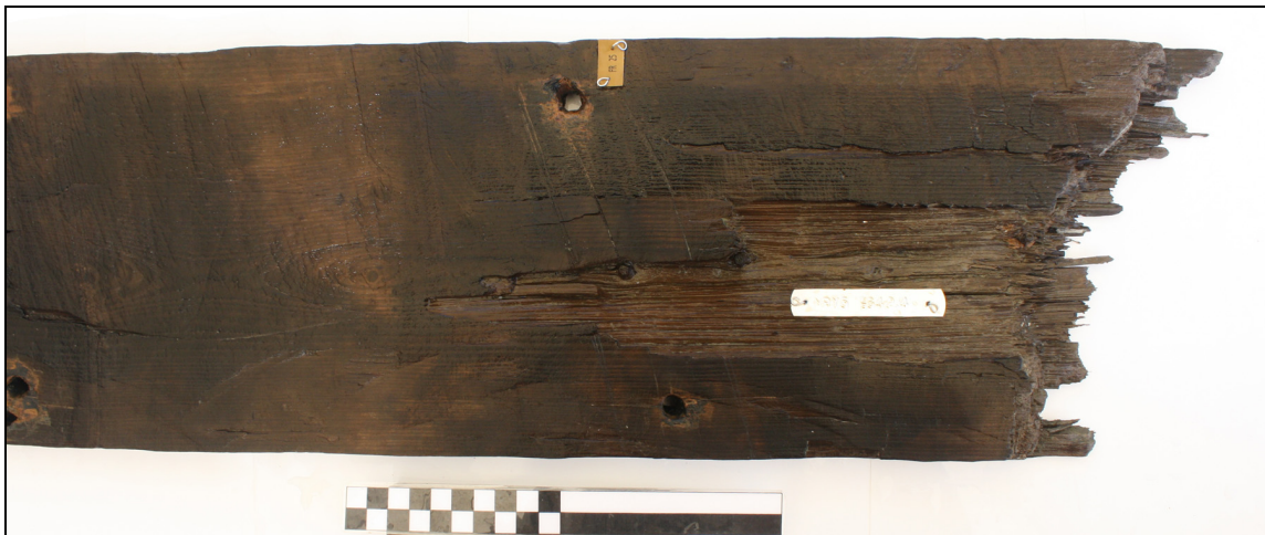
Figure 4.97. Charred areas on the inner face of SS 4-2 at FR 25.
