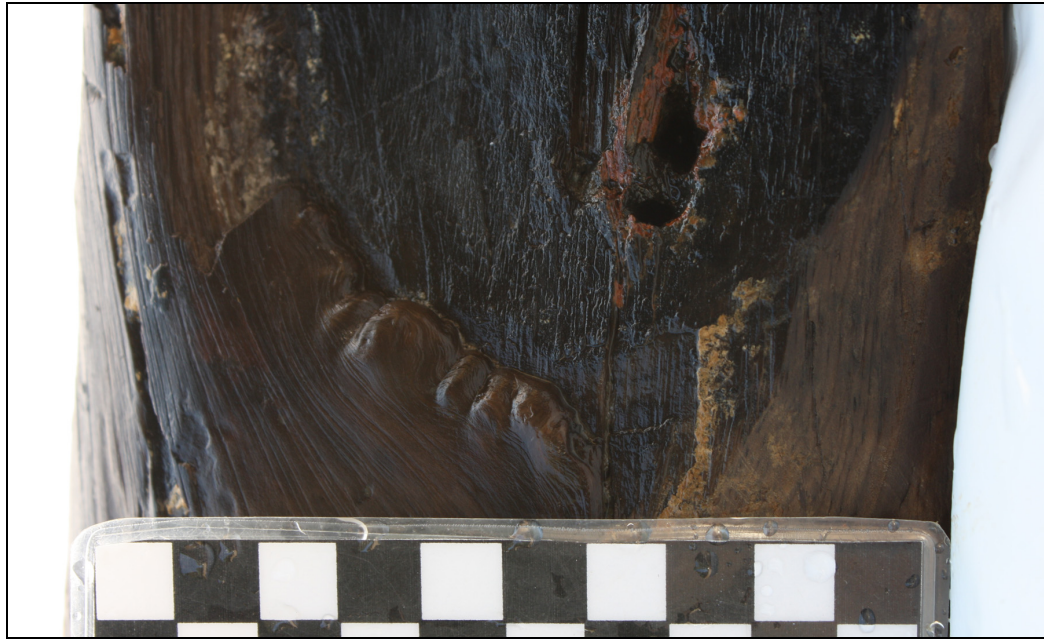
Figure 4.29. Fire scarring on the outer face of FR 11.
