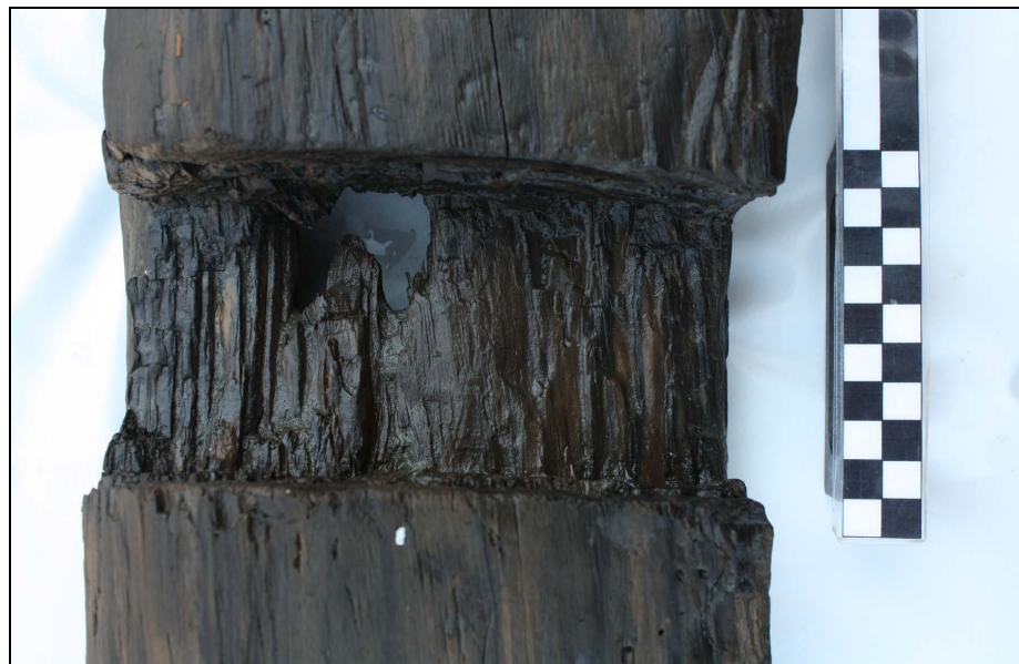
Figure 4.168. Rough edges of mortise on outer face of S-Block 4.
