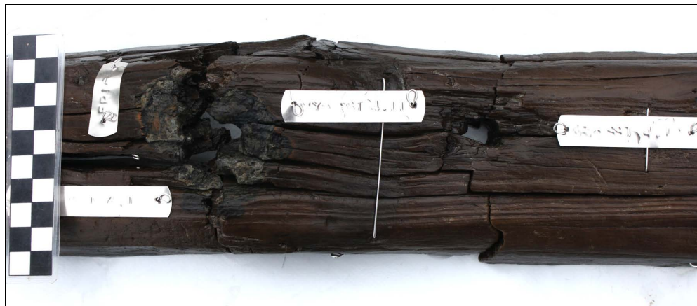
Figure 4.133. Inner face of SST 4 at FR 16. Note difference between used (to left) and disused (to right) nail holes.
