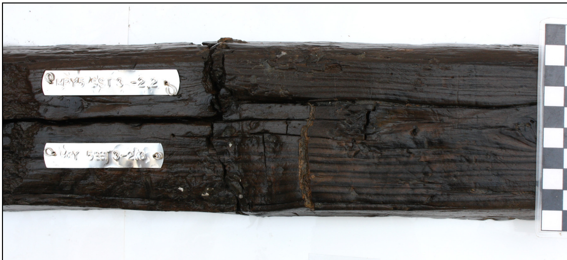
Figure 4.125. Pitched crack on the inner face of SST 3-2 at FR 21.
