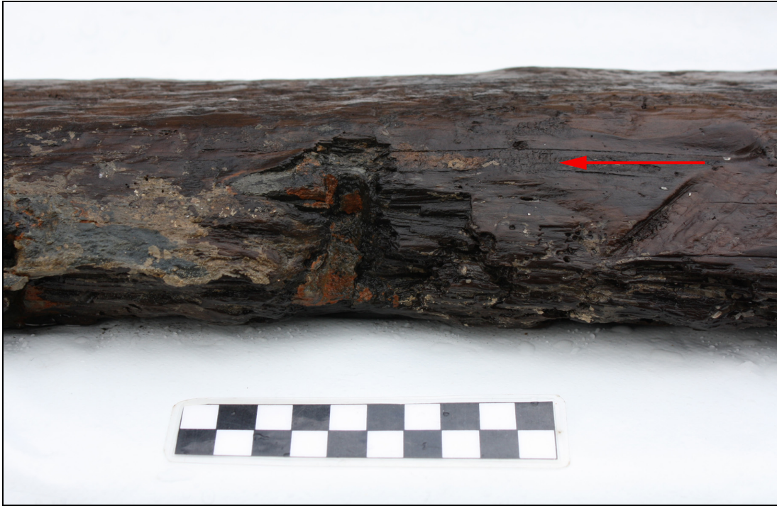
Figure 4.112. Wale SS 13 top edge at FR 7-FR 8. Iron nail hole and pitch outline (red arrow) indicate a through-beam at this location.
