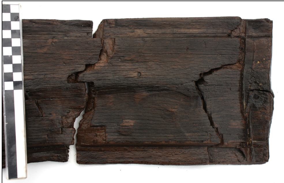
Figure 4.151. Outer face of recycled ceiling plank SC 1B, forward end. Note deep groove along damaged edges and compression damage at end.
