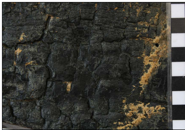
Figure 4.98. Charred inner face of PS 3-1 at FR 3-FR 4.
