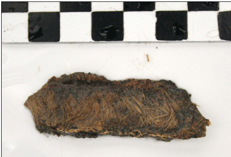
Figure 4.91. Caulk removed from top edge of PS 2-4 at FR 20-FR 21.
