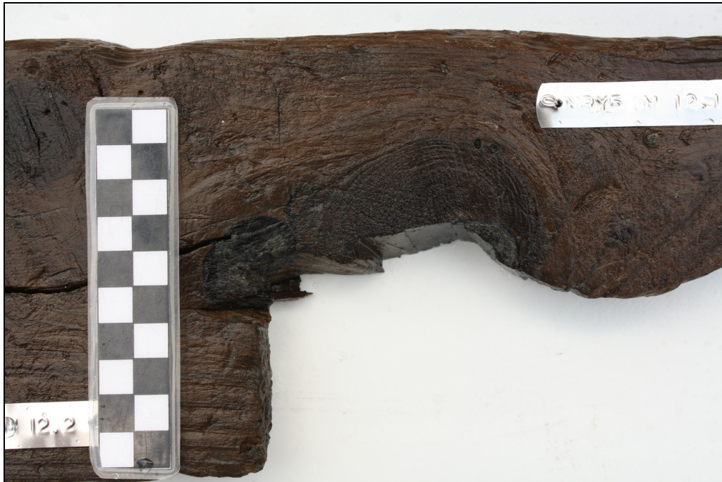
Figure 4.158. Upper face of UM 12, showing roughly chiseled recess at timber forward of F 13.
