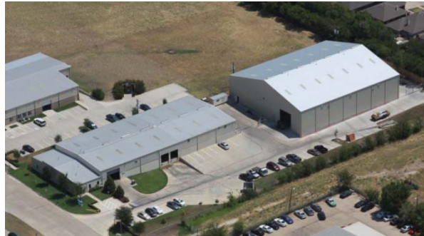
Fig 1.1: Aerial view of Isotherm, Inc. in Arlington, Texas
