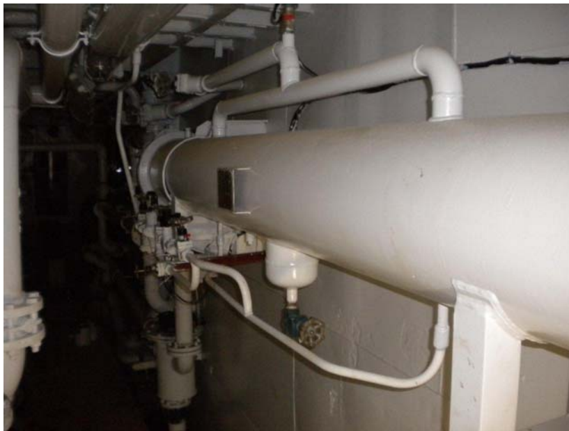
Fig. 2.13: One of the two installed SX chillers on a trawler in Ecuador
