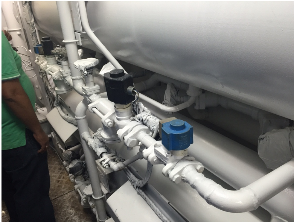
Fig. 2.17: Correct dual valves AKVA installation on an SX Chiller in a Master/Slave configuration
