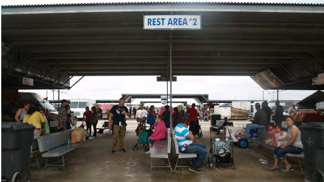
Figure 4.40: Typical Rest Area at Cameron County Market Source: Photo by Author, 2015
