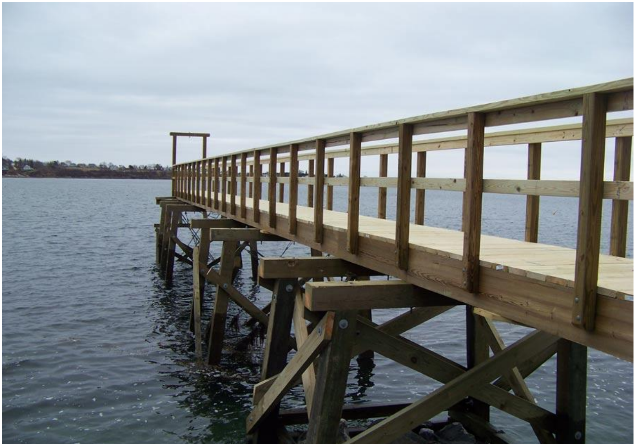
Figure 3: Typical pier made of timber
