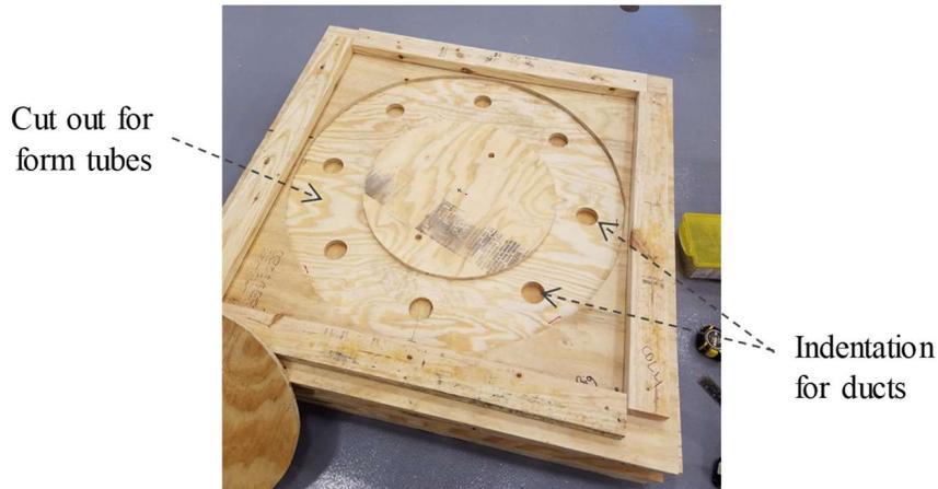
**Figure 4-19. Column segment formwork: bottom plate**
