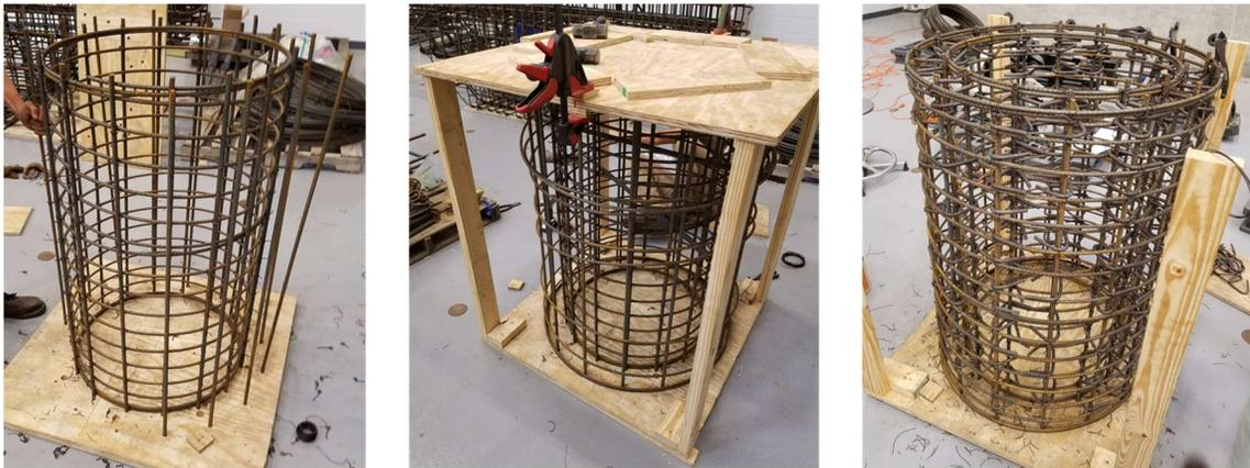
**Figure 4-17. Building reinforcement cages for column segments**
