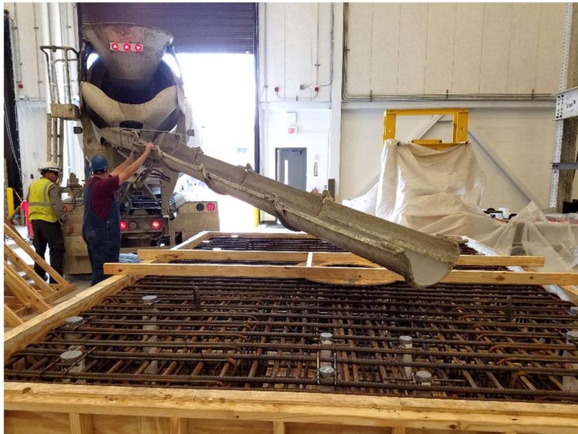
**Figure 4-34. Concrete casting of foundation block**
