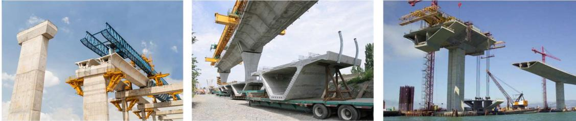
**Figure 1-1. Precast concrete segmental bridge construction**
