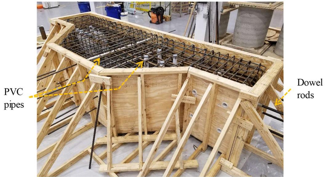
**Figure 4-28. Formwork of loading beam before concrete casting**
