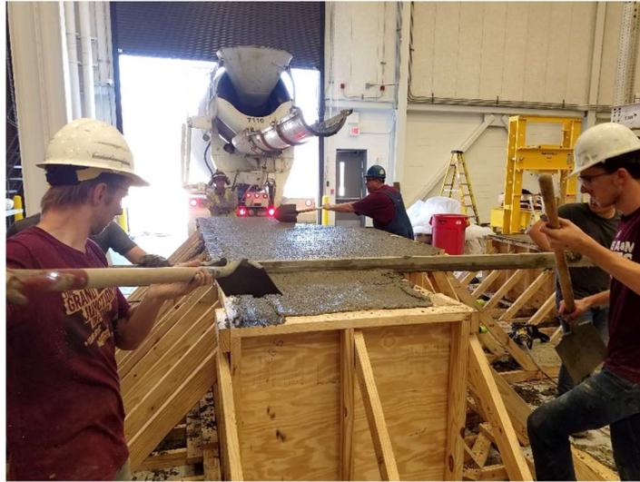
**Figure 4-30. Concrete casting of loading beam**
