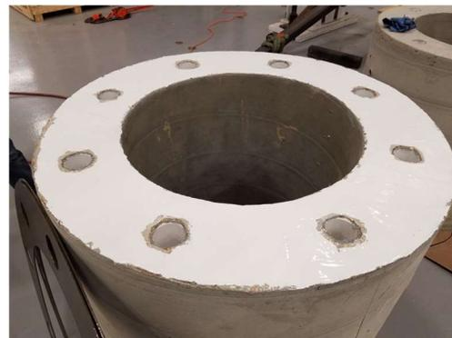
**(2) Application of epoxy on concrete surface**
