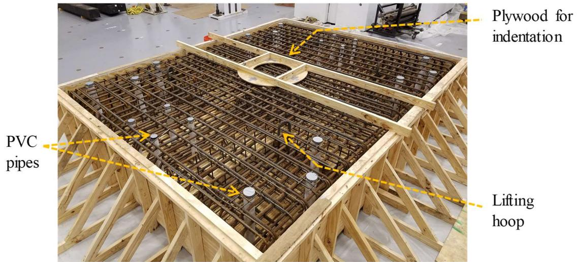
**Figure 4-33. Formwork of foundation block before concrete casting**
