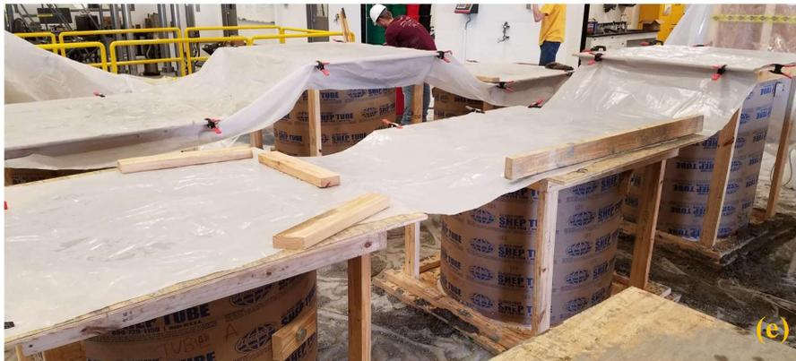
**Figure 4-22. Casting of column segments: (a) ready mixed concrete delivery by truck; (b) pouring concrete in forms; (c) compaction by vibrator; (d) surface finishing; (e) covering forms for curing**
