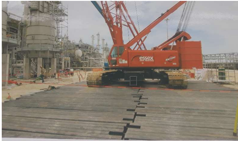
Figure 1 Example operation of construction mat
