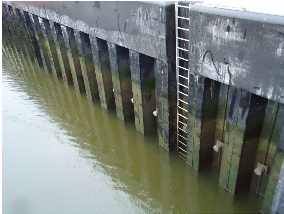
Figure 4 Contemporary port/harbor installation, quay wall
