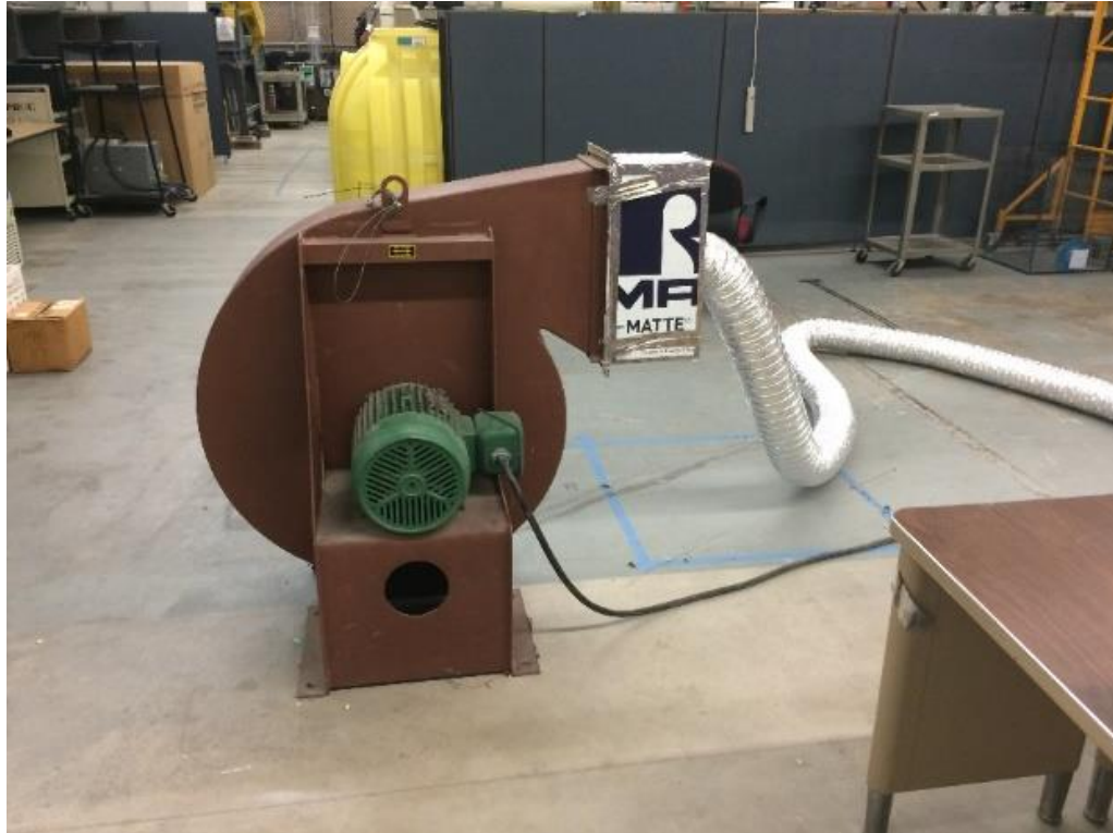
Figure 11. New blower used with aluminum duct to reach inlet
