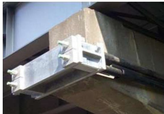
(b) Morrison Avenue bent cap
