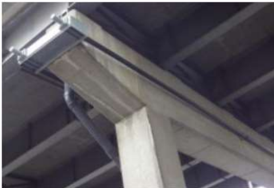
(a) Hawthorne Avenue bent cap
