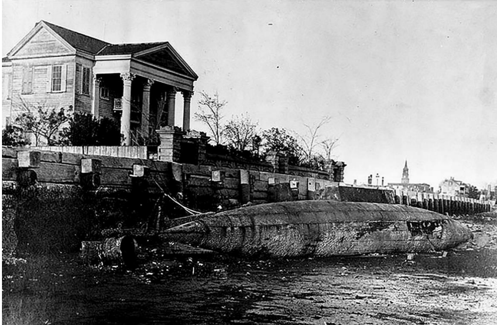
Figure 34. A "David" abandoned on the dock at low-tide on Tradd Street. Naval History and Heritage Command, Washington, D. C., Photo#165-C-752.
