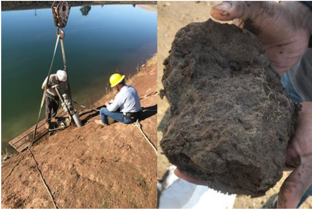
Figure 5.1 Soil sampling operation at a lime treated section of the FKC
