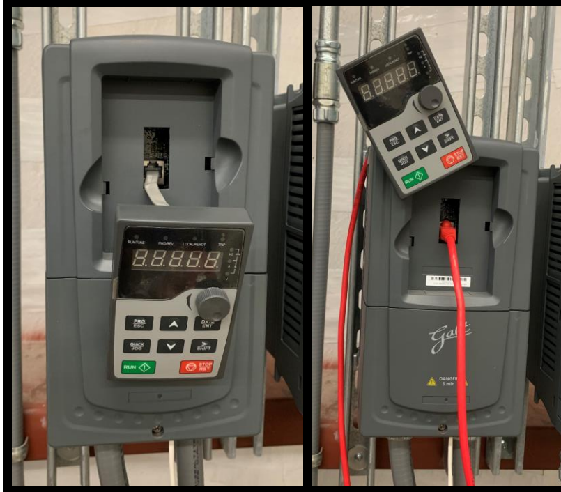
Figure 3.20: VFD before (left) and after (right) the cable extension.
