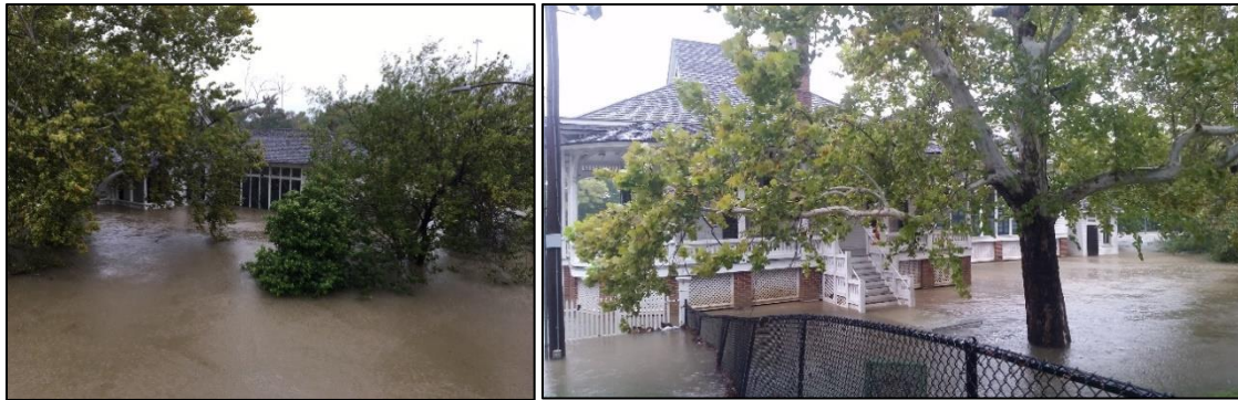
Figure 61 The historic 1868 Pillot House in Sam Houston Park, Houston, flooded by Hurricane Harvey. Photos courtesy of Ginger Berni.
