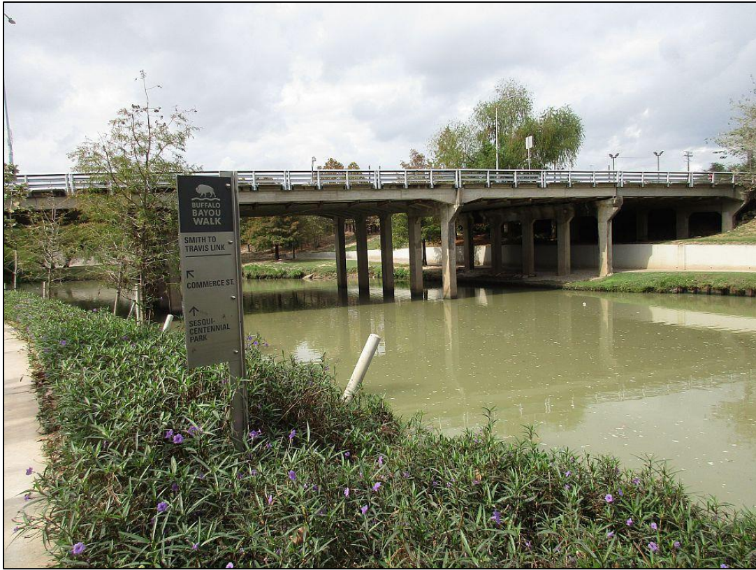
Figure 16 The Milam Street Bridge, Houston, Texas in 2015. Photo courtesy Linda Gorski.
