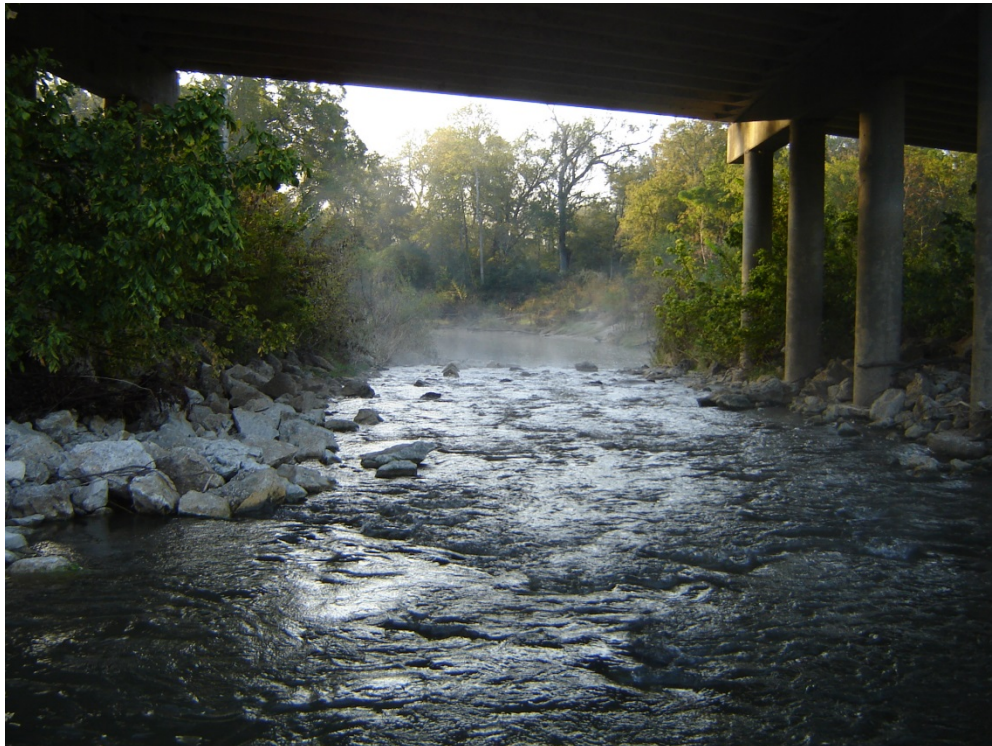
Carters Creek under bridge downstream of William D. Fitch
