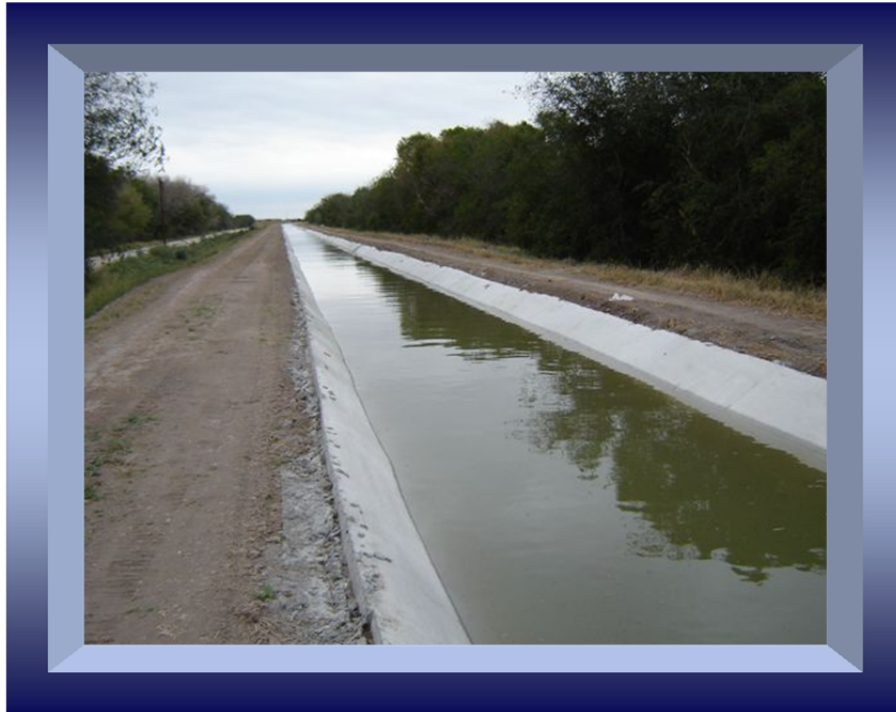
Figure 6: Example of Lined Canal
