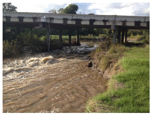
High flow event on Carters Creek at WM D. Fitch Pkwy (Station 21259) in October 2013. Events such as this have caused severe erosion at this site as is evidenced by the near vertical creek bank on the right side of the photo.
