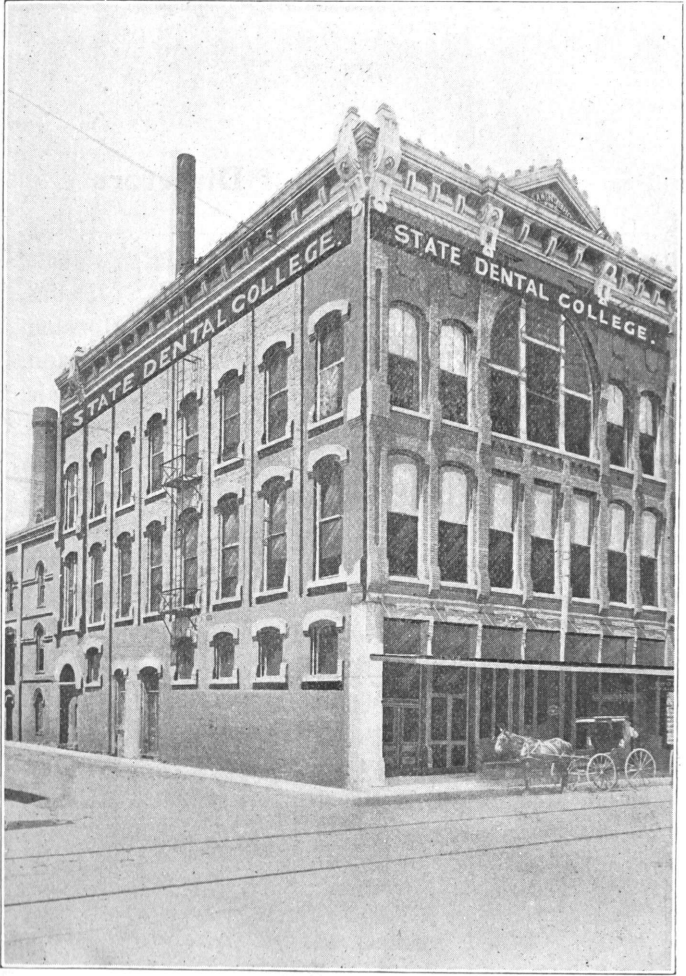
New College Building, 437 South Ervay
