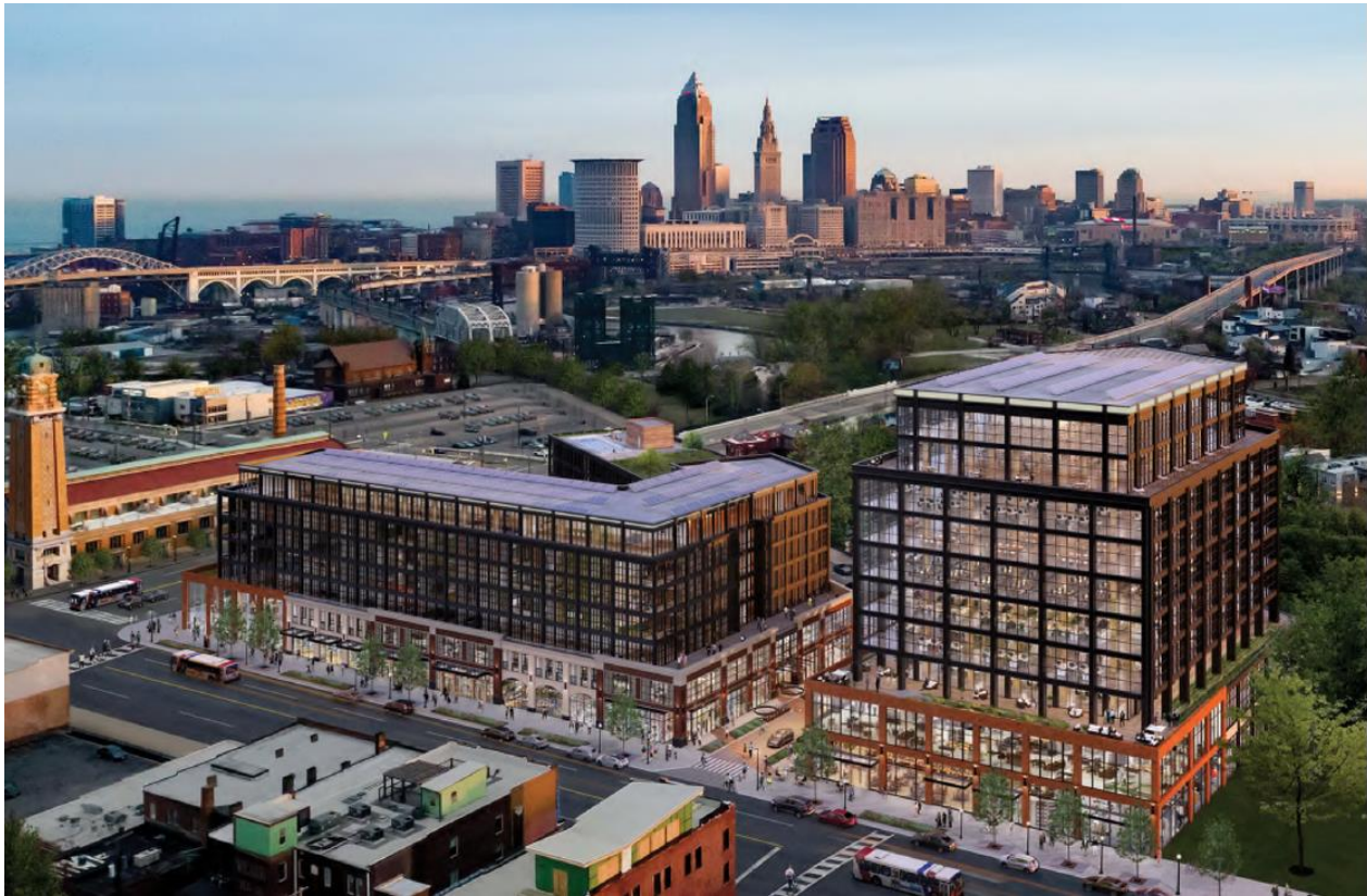
Figure 1.1: Image of the proposed Market Square project showing the possible photovoltaic (PV) panel installation.
