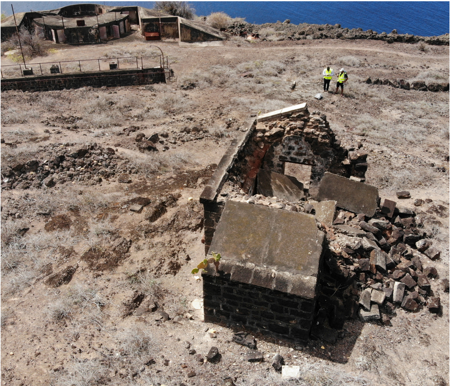
Figure 11: Oblique aerial view of ruined structure at West Munden's Hill (Image: B. Fortenberry).
