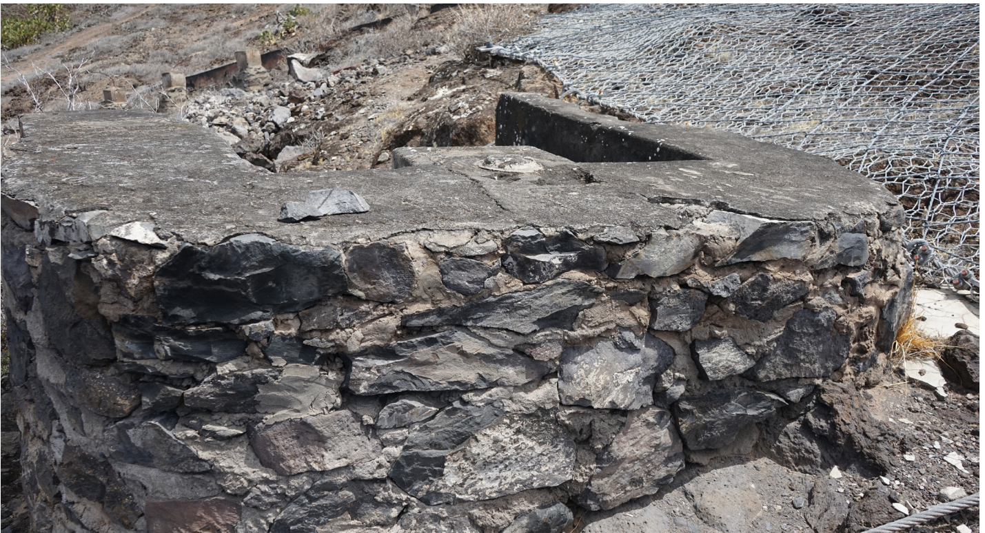
Figure 16: Detail view of surviving firing position at East Munden's Hill (Image: B. Fortenberry).
