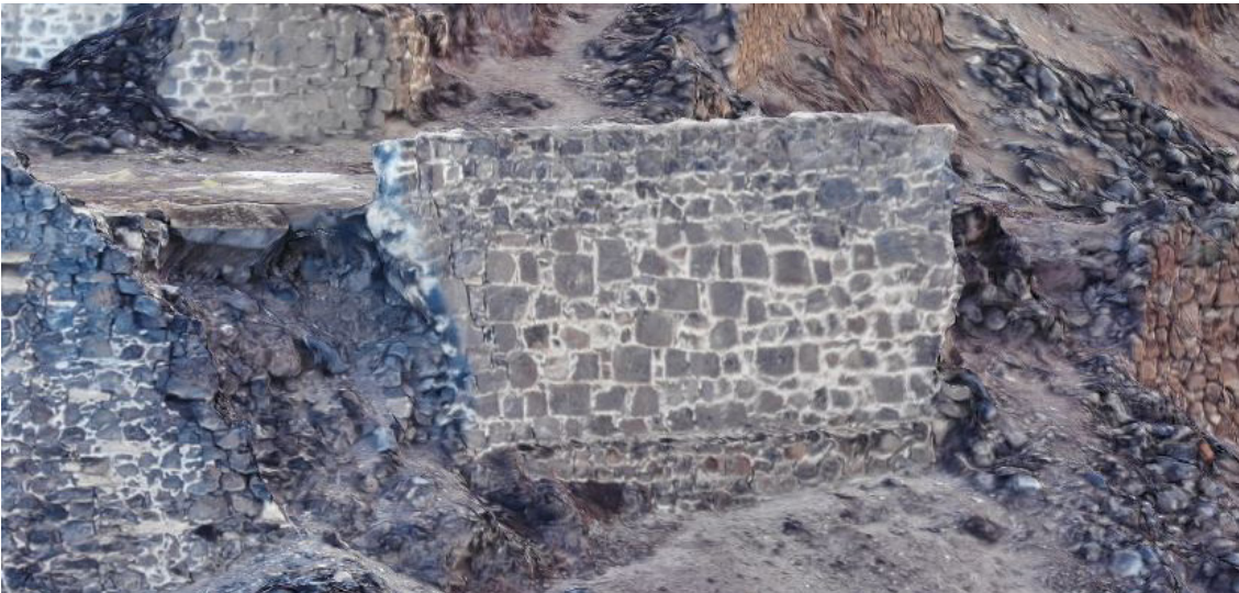
Figure 9: Photogrammetric model, detail of wall collapse at Upper Banks' (Model: B. Fortenberry).
