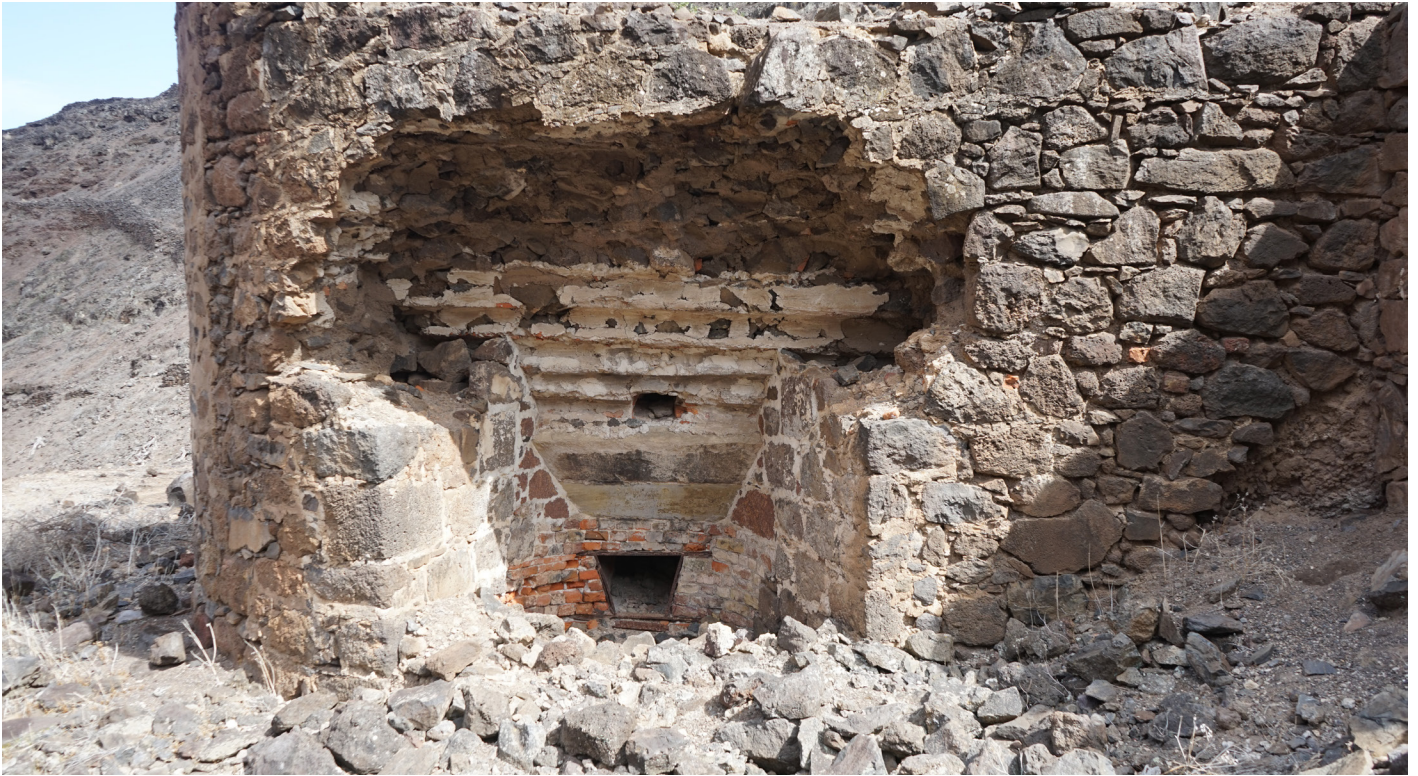
Figure 61: Detail of firing hole of lime kiln (Image: B. Fortenberry).
