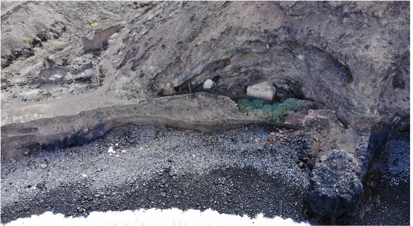
Figure 25: Aerial image of surviving fabric at East Munden's Hill looking southwest (Image: B. Fortenberry).
