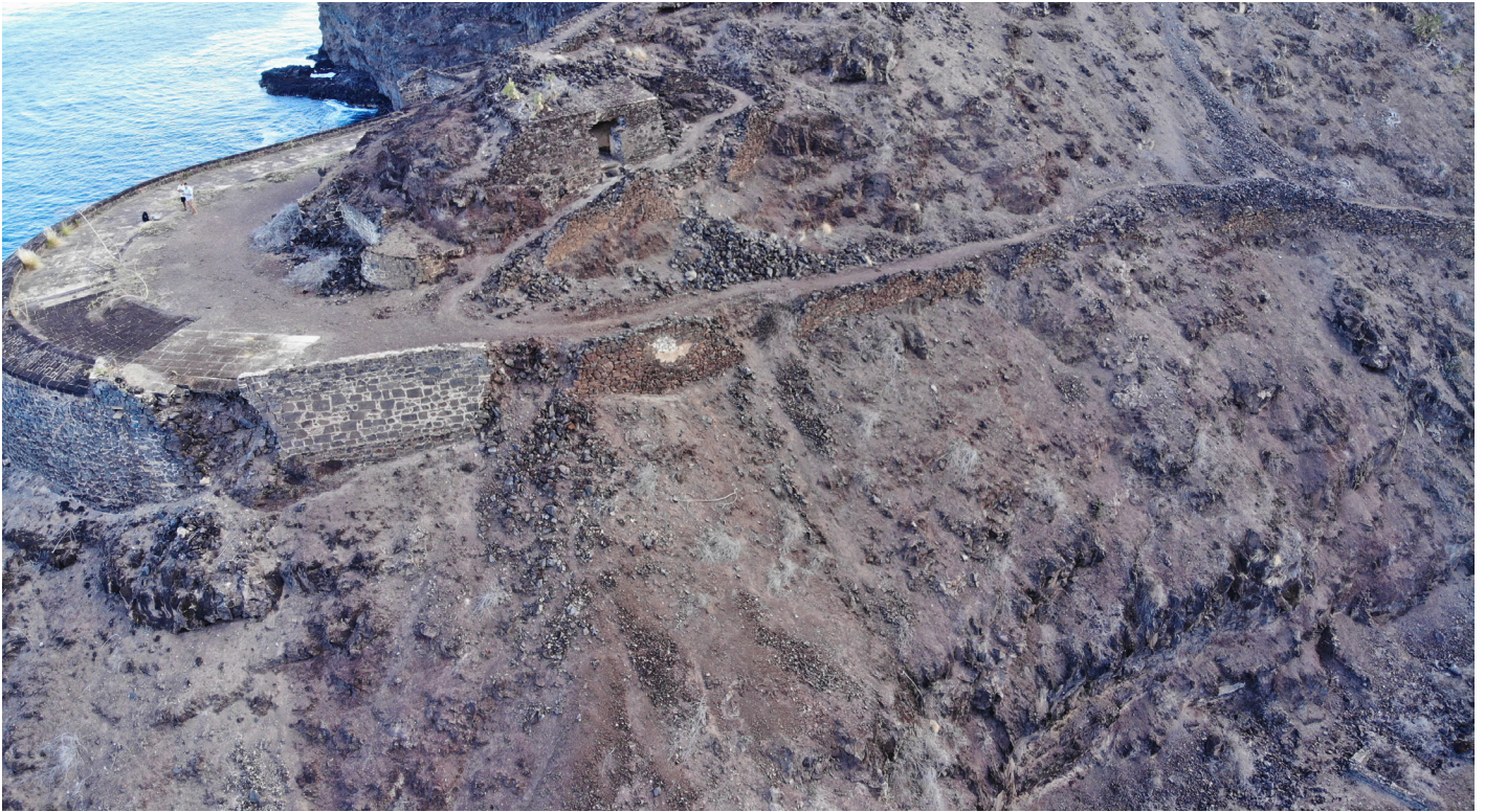
Figure 48: Oblique aerial view of wall collapses on the south side of Upper Banks' Battery (Image: B. Fortenberry).
