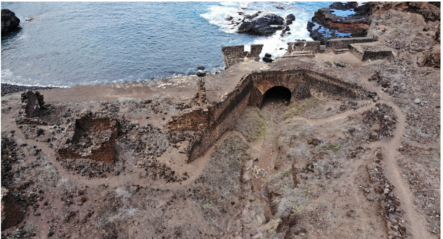
Figure 14: Lower Banks' Curtain Wall and Ruined Support Structures (Image: B. Fortenberry).
