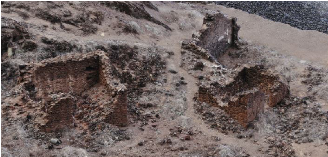
Figure 9: Photogrammetric model, ruined barracks and support buildings at Lower Banks' Battery (Model: B. Fortenberry).
