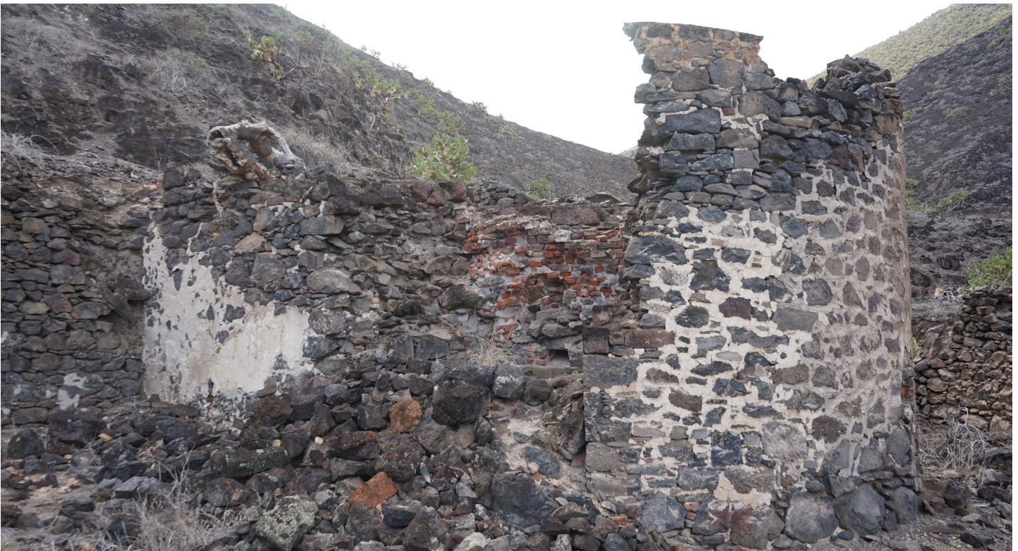
Figure 62: Ruined west wall of Lower Banks' Lime Kiln. (Image: B. Fortenberry).
