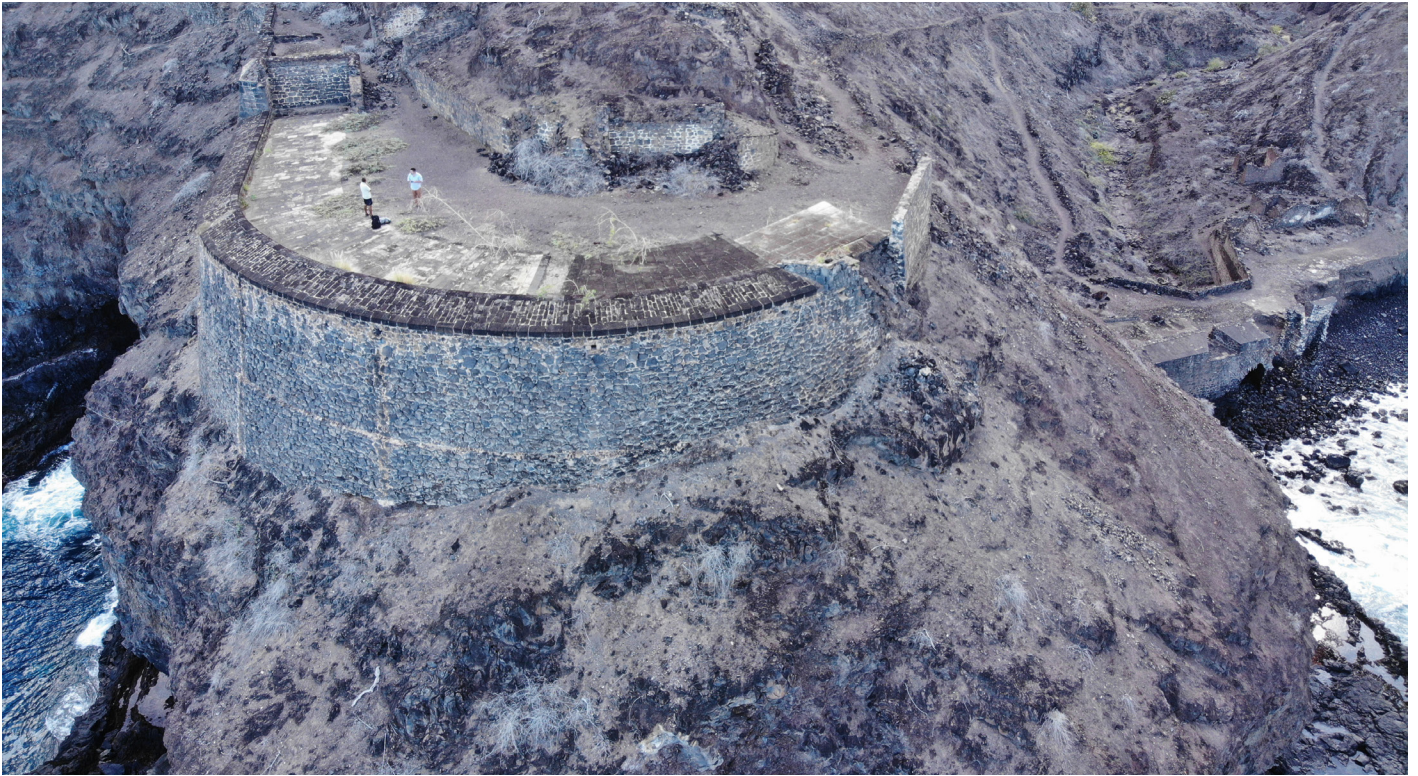
Figure 38: Oblique aerial view of Half Moon Battery at Upper Banks' Battery looking east (Image: B. Fortenberry).
