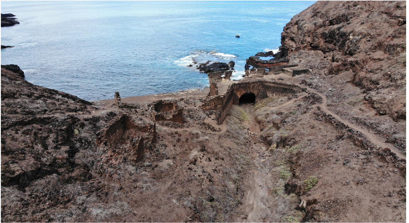
Figure 13: Lower Banks' Curtain Wall as viewed from the east (Image: B. Fortenberry).
