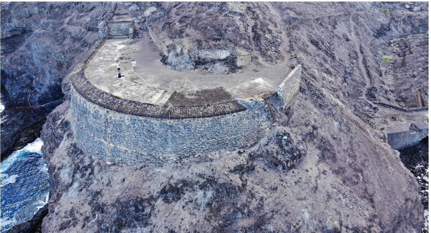
Figure 39: Oblique aerial view of Half Moon Battery at Upper Banks' Battery looking east, southern wall collapse in partial view (Image: B. Fortenberry).
