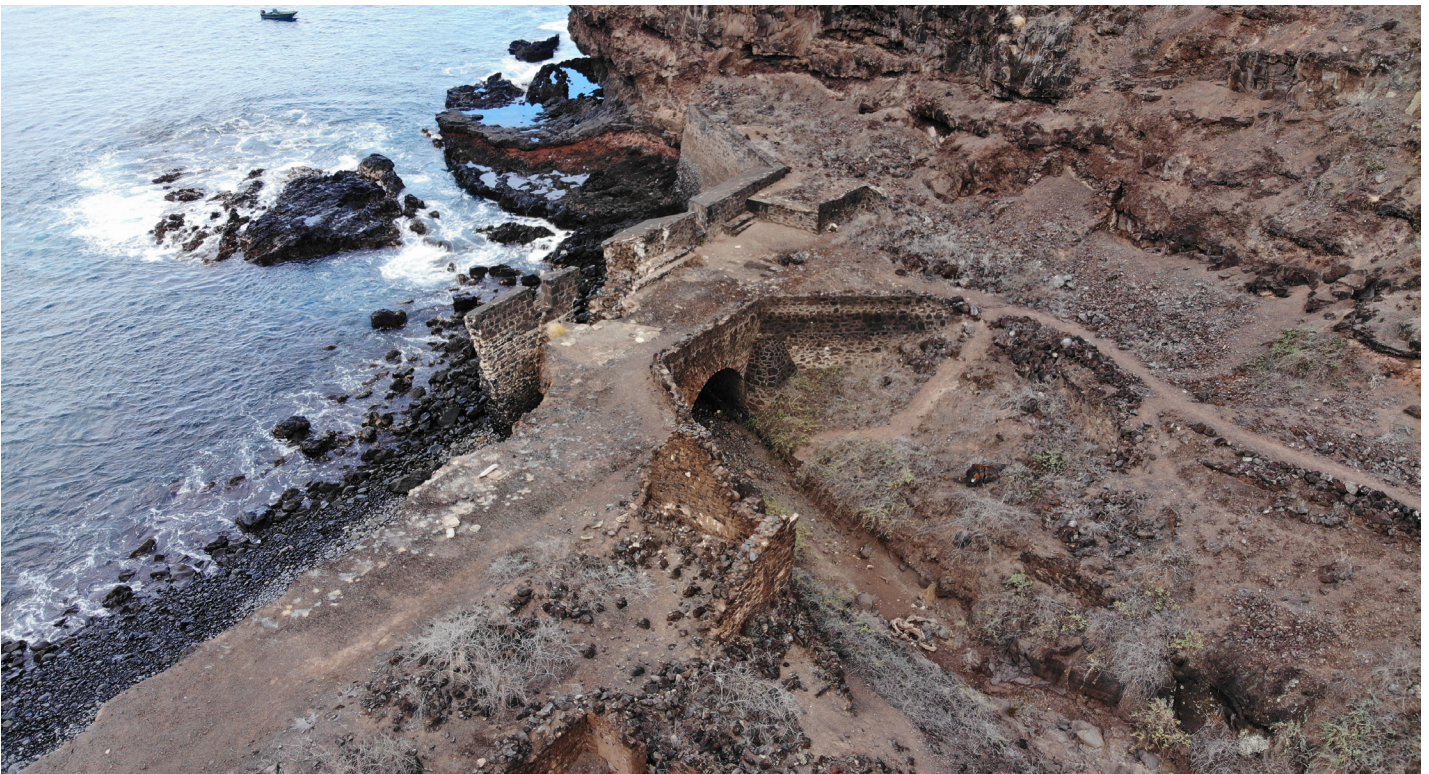
Figure 18: Aerial image of curtain wall Lower Banks' Battery (Image: B. Fortenberry).
