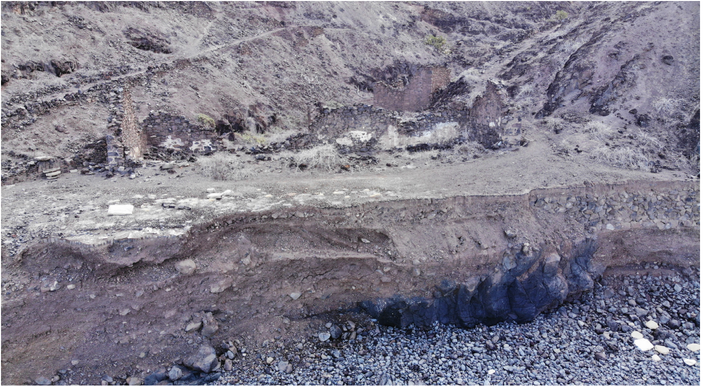
Figure 27: Detail aerial image of support buildings looking east at Lower Banks' Battery (Image: B. Fortenberry).
