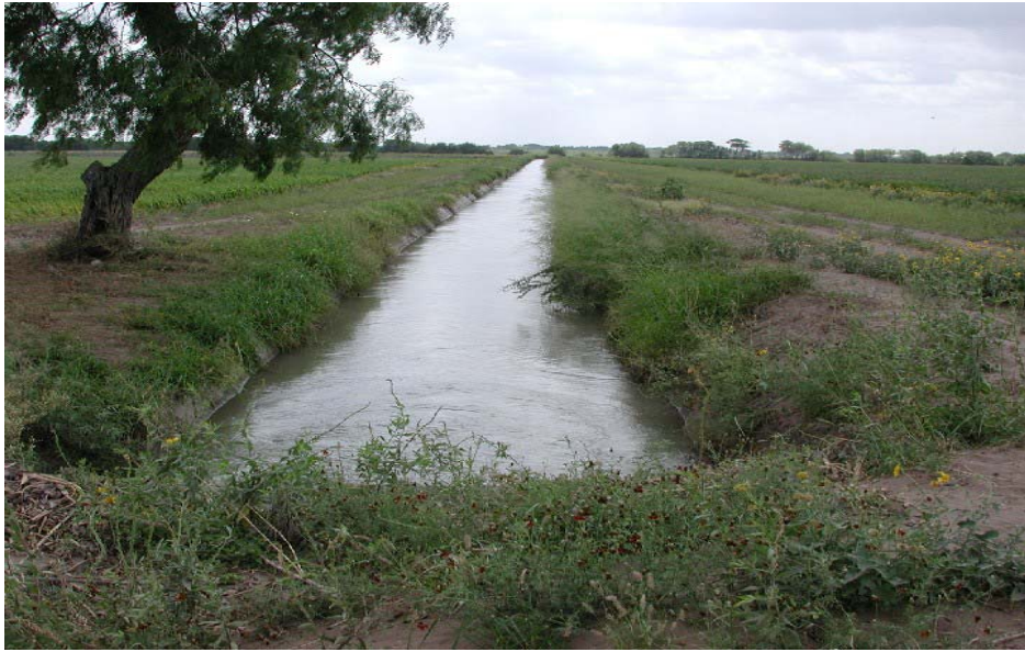
Figure 4. Canal 13's flow measurement location.
