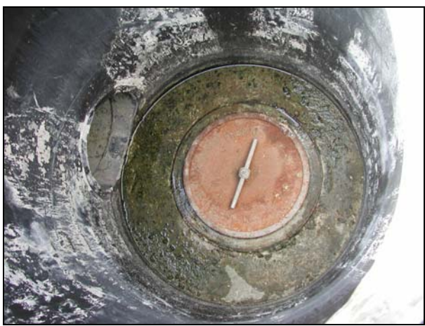
Figure 6. Typical 14-inch Fresnos alfalfa valve used in the district.
