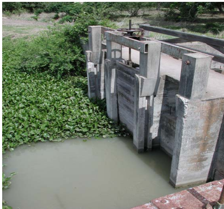
Figure 1. Head gate inlet into canal B (one operational gate).
