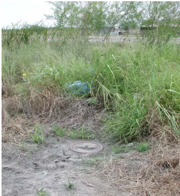
Figure 11. Farm turnout valve at canal 27 and B.
