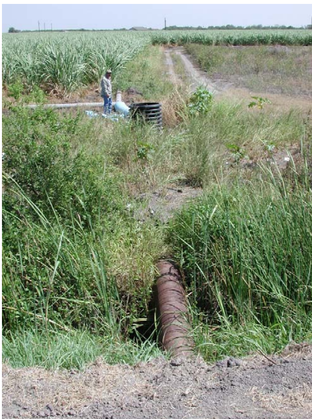
Figure 7. A typical 15-inch steel pipe feeding a black poly-riser, usually fitted with a 12-inch pipe outlet feeding into poly-pipe.
