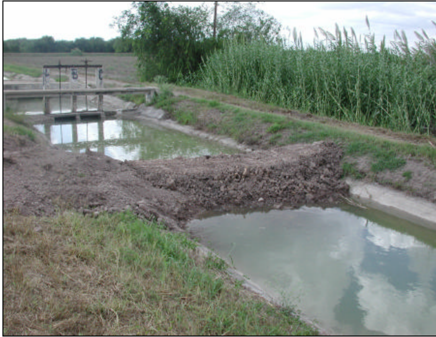
Figure 2: Earthen dam constructed on Lateral A - Stewart Rd.
