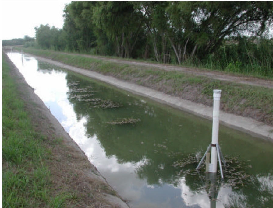
Figure 3: Continuous-stage level recorders on Lateral A - Stewart Rd.
