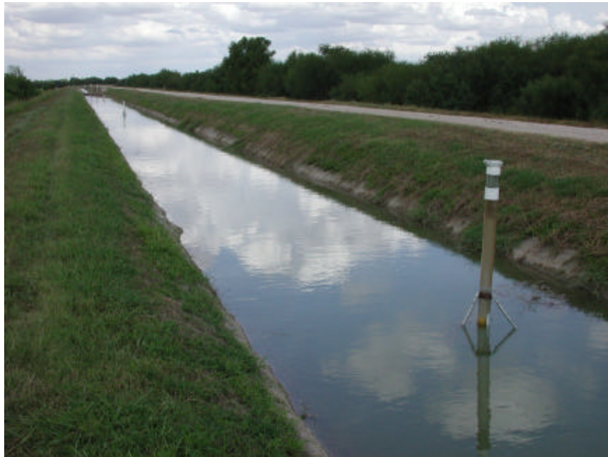
Figure 9: Continuous stage level recorders on Lateral A – I Rd.
