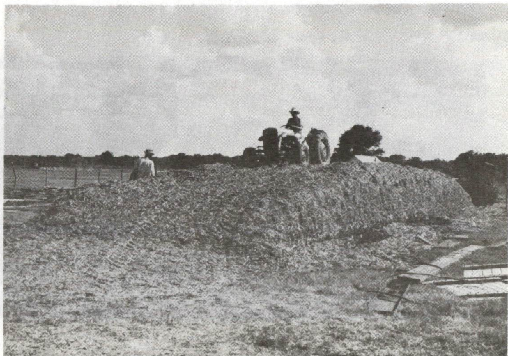
Figure 8-1. Stack silos were formed by stacking silage directly on the ground or on a concrete slab. A minimum width of 16 feet is recommended.
