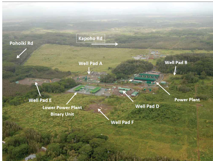
Figure 3.2: Areal View of the Puna Venture Power Plant (adapted from ORMAT)
