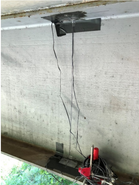
(a) Example of Installed Strain Gauges
