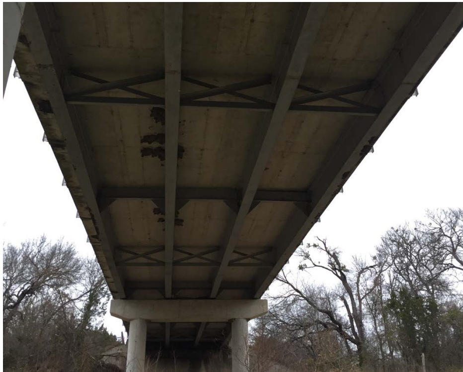
(b) Underside view
