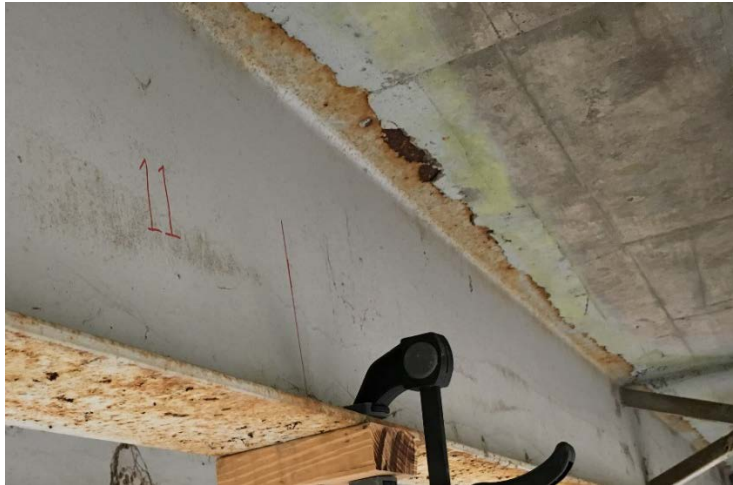
Figure 7.3. Observation of Girder Flange Embedment with No Signs of Cracking
