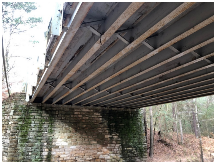
(b) Underside view
