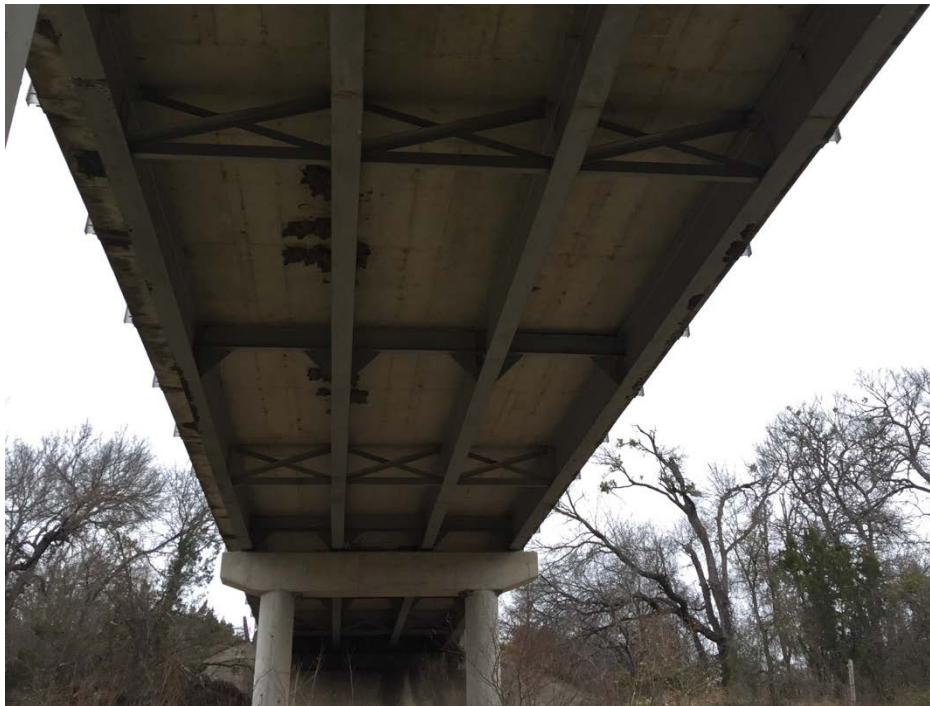
(b) Underside view
