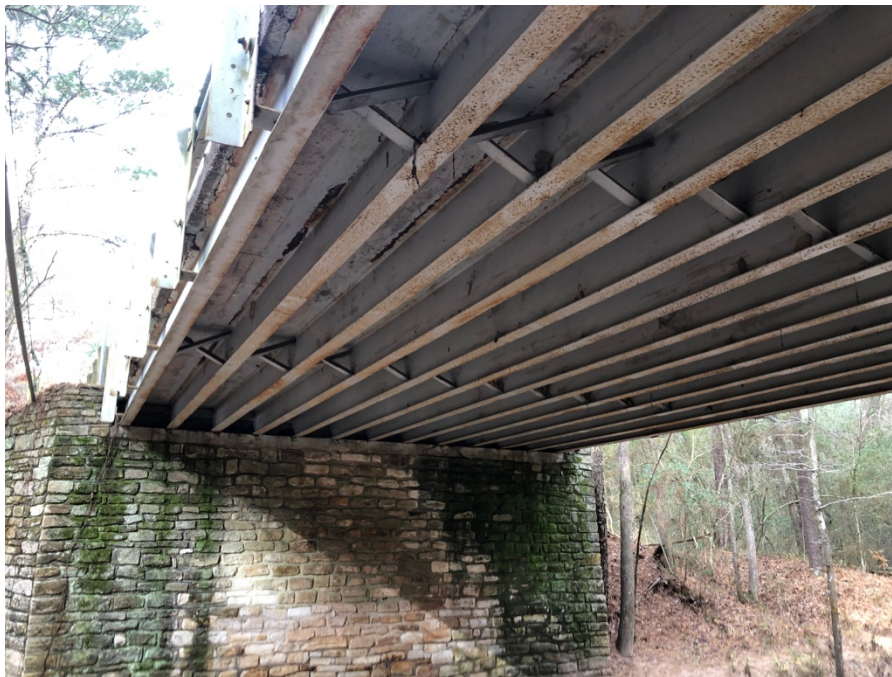
(b) Underside view
