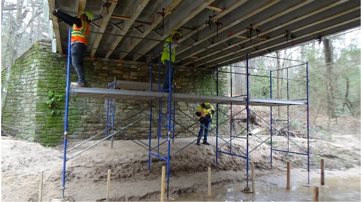
(a) Instrumentation of Bridge SM-5
