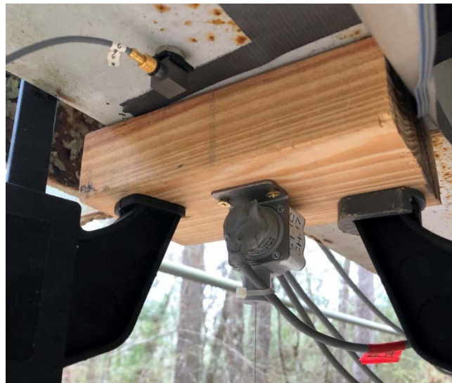
(b) Installed String Potentiometer and Accelerometer at Midspan of a Girder
