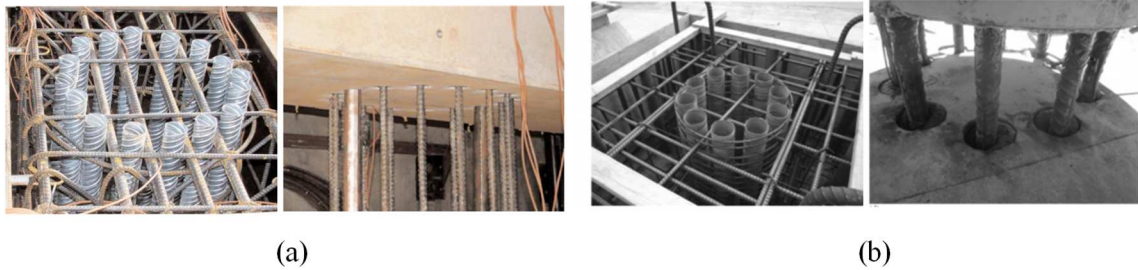
Figure 1.3. Grouted duct column connection: (a) Restrepo et al. (2011); (b) Tazary and Saiid Saiidi (2015)).
