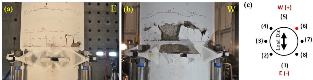
Figure 7.67. Damage state in PUED-2 column at 1.8×DE (1.2×MCE) at the loading rate of 2.71 in/sec (0.025 drift ratio/sec): (a) cover concrete spalling on east side; (b) cover concrete spalling on west side; (c) location of fractured ED link (red circle).
