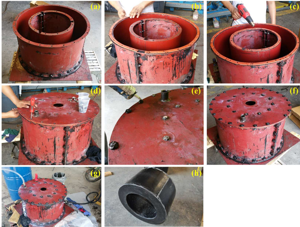
Figure 7.28. Casting of PU sleeve: (a) mold shells bolted to the base plate; (b) sealing the top interface; (c) heating the silicone sealant; (d) bolting the top lid; (e) sealing bolted connections; (f) final mold assembly prior to casting; (g) injecting the PU material solution; (h) PU sleeve after demolding.
