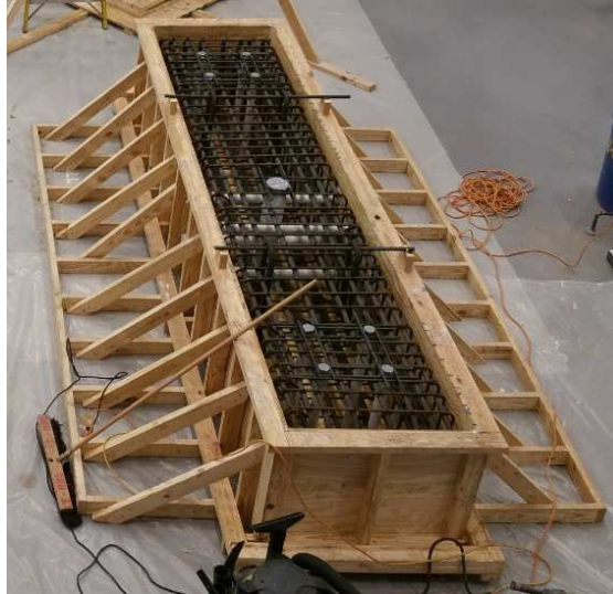
Figure 7.24. Cap beam reinforcement cage in the formwork: final assembly.
