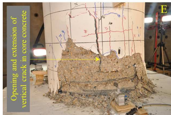
Figure 7.39. Damage in RC rocking column at 11.09% drift ratio: opening of vertical crack in the core concrete on east side.
