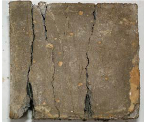
(b) Crack pattern observed experimentally under uni-axial compressive loading in the vertical direction [66]
