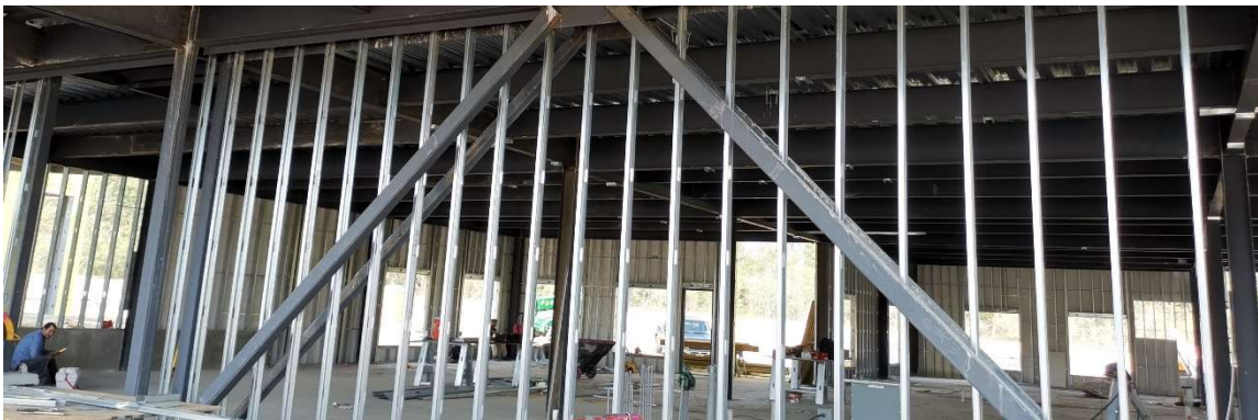
Figure 25 The small-size structure like steel structure
