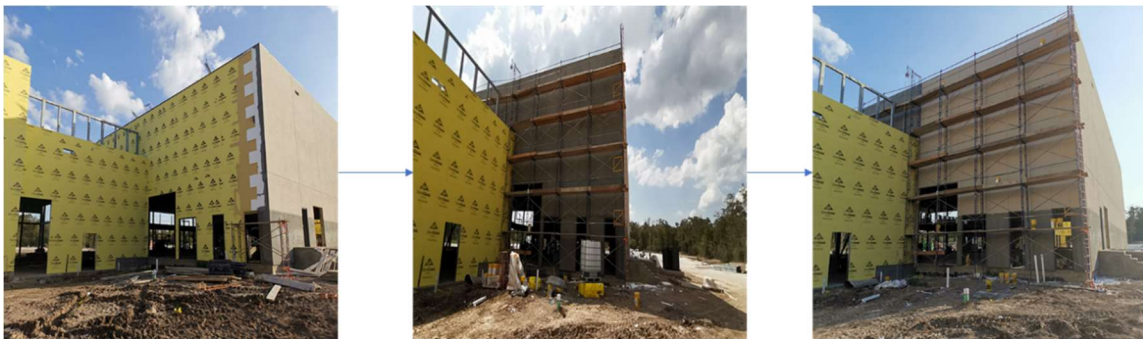
Figure 9 The construction process of the external wall
