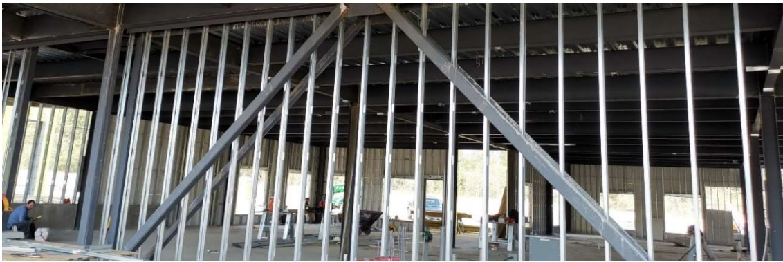
Figure 25 The small-size structure like steel structure
