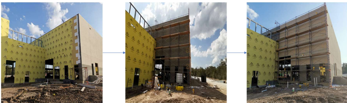
Figure 9 The construction process of the external wall
