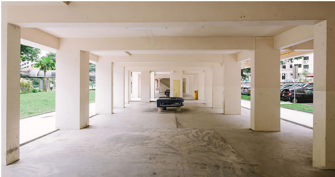
Figure I-10. Example of typical ground floor setting in public housing buildings.
