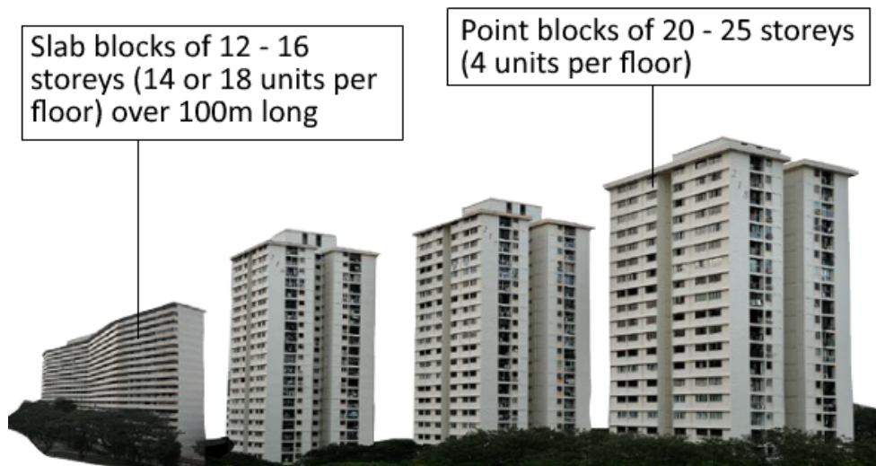
Figure I-7. Typical public housing typology in Singapore built between the 1960s to 1980s, constituting 80% of existing public housing.
