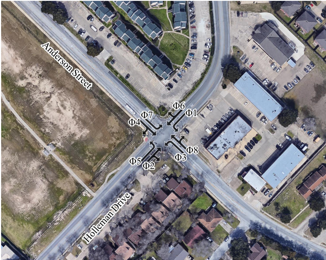
Figure 9. Anderson Street (minor street) at Holleman Drive (major street) in College Station, Texas.
