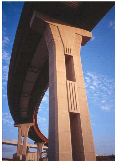
Figure 2.4 Steel Twin Tub Girder Bridge I 35/US 290 Interchange, Austin, Texas (Reprinted from Coletti 2005)
