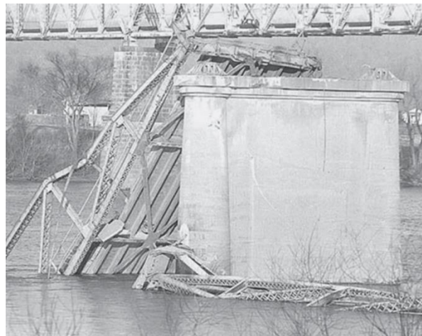
Figure 2.1: Silver Bridge after the collapse in 1967 (Reprinted from NTSB 1971)
