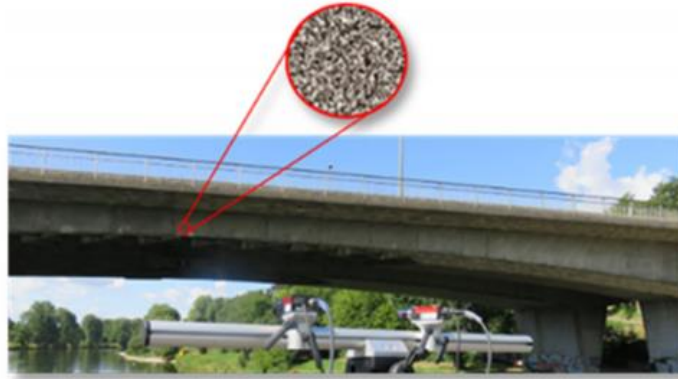
Figure 6. DIC assessment of bridge courtesy of Dantec Dynamics. Used with permission [18].
