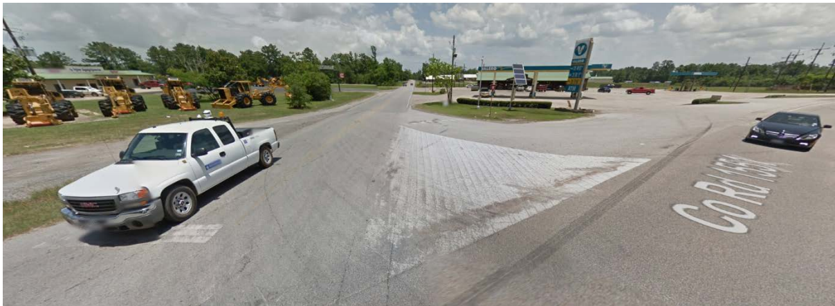
Figure 14: Low Visibility of Road Markings at Intersection 3
