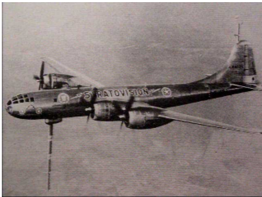
Fig. 2. Stratovision B-29 research aircraft with TV transmit antenna extended below aircraft (photo courtesy of the Early Television Museum). Photo reprinted from [8].
