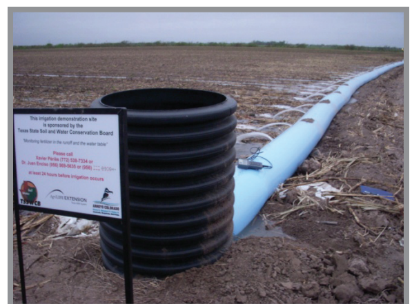
Figure 1: Irrigation poly pipe utilized during an irrigation event
