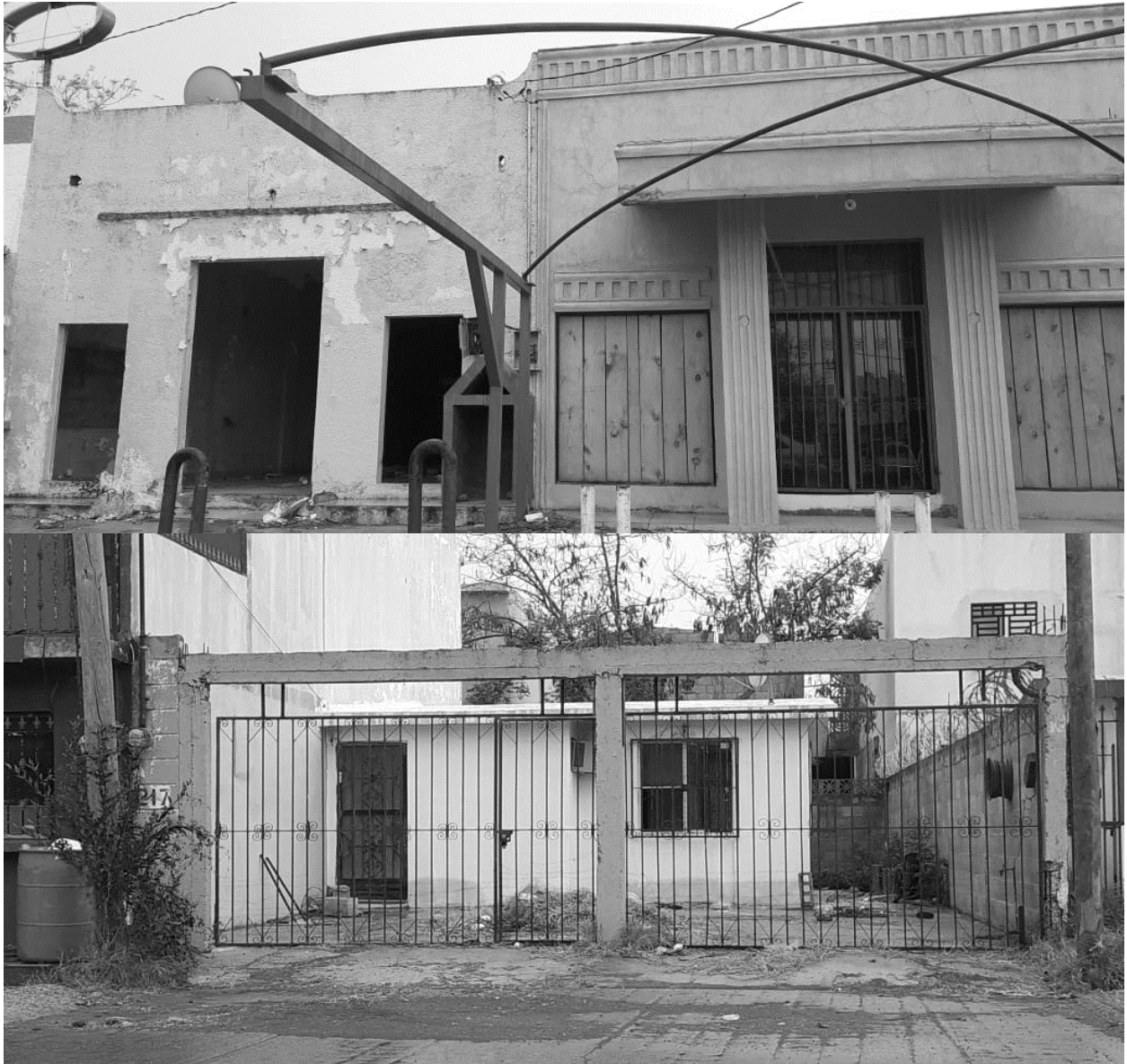
Figure B-6 Own Photographs. Abandoned Housing: Colonia Roma, Reynosa, Tamaulipas, Mexico (2019).
