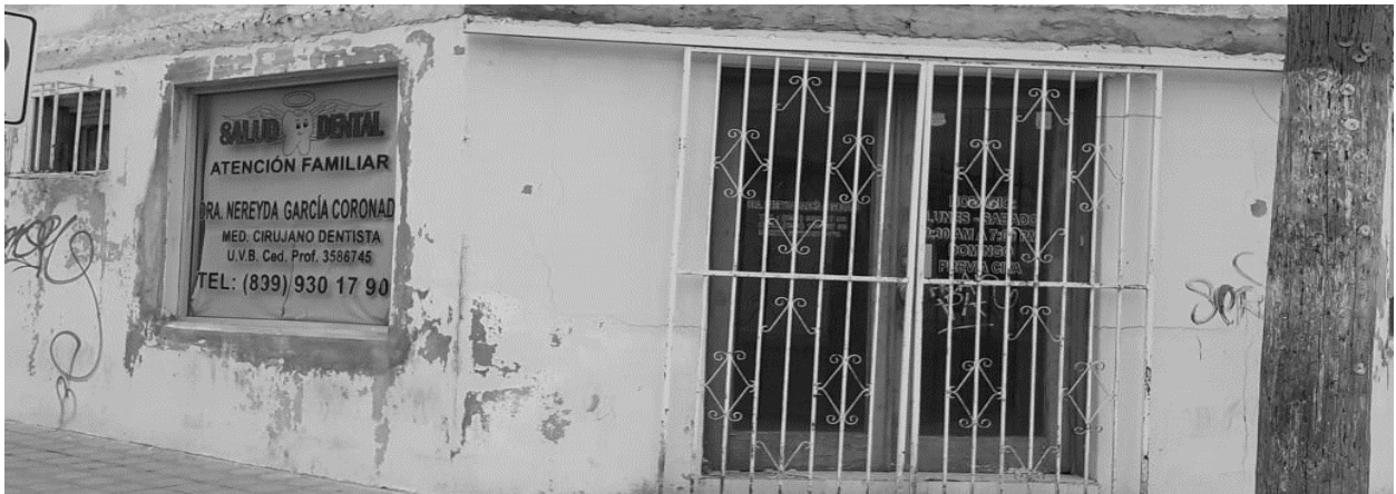
Figure B-3 Own Photographs. Abandoned Housing: Zona Centro, Reynosa, Tamaulipas, Mexico (2019).
