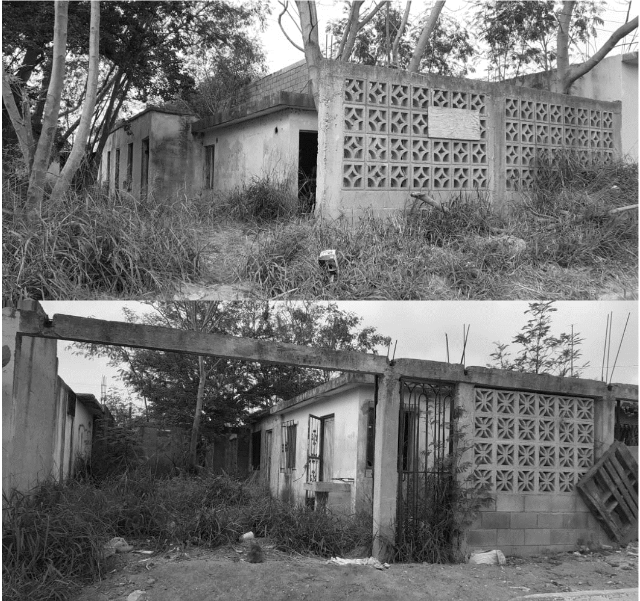
Figure B-9 Own Photographs. Abandoned Housing: Colonia Mexico, Reynosa, Tamaulipas, Mexico (2019).
