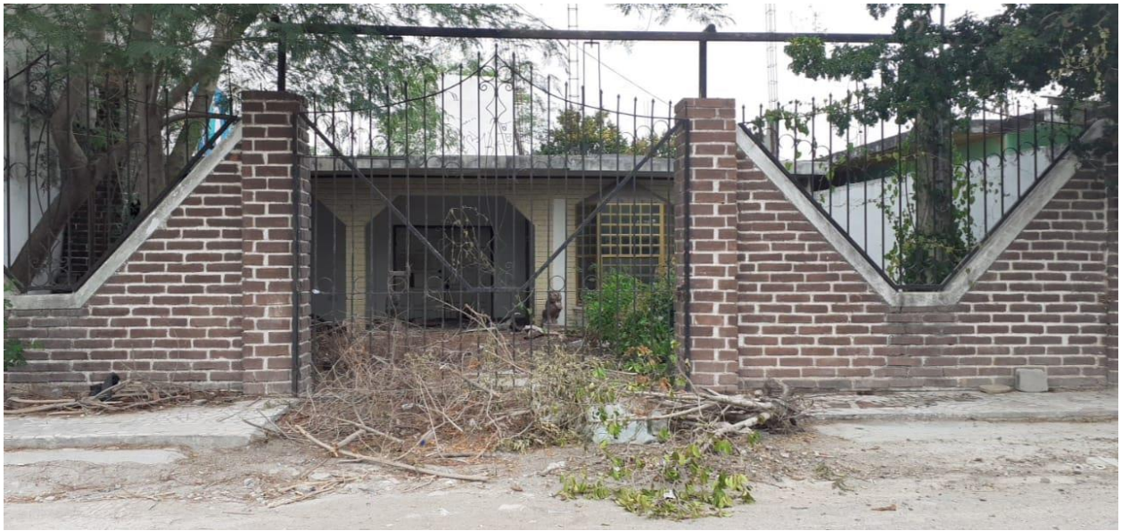
Figure B-7 Own Photographs. Abandoned Housing: Colonia Roma, Reynosa, Tamaulipas, Mexico (2019).
