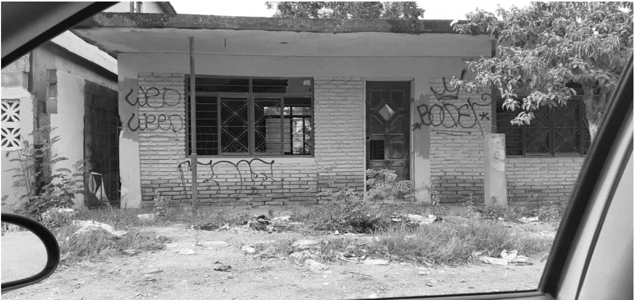
Figure B-14 Own Photographs. Abandoned Housing: Colonia Naranjitos, Reynosa, Tamaulipas, Mexico (2019).
