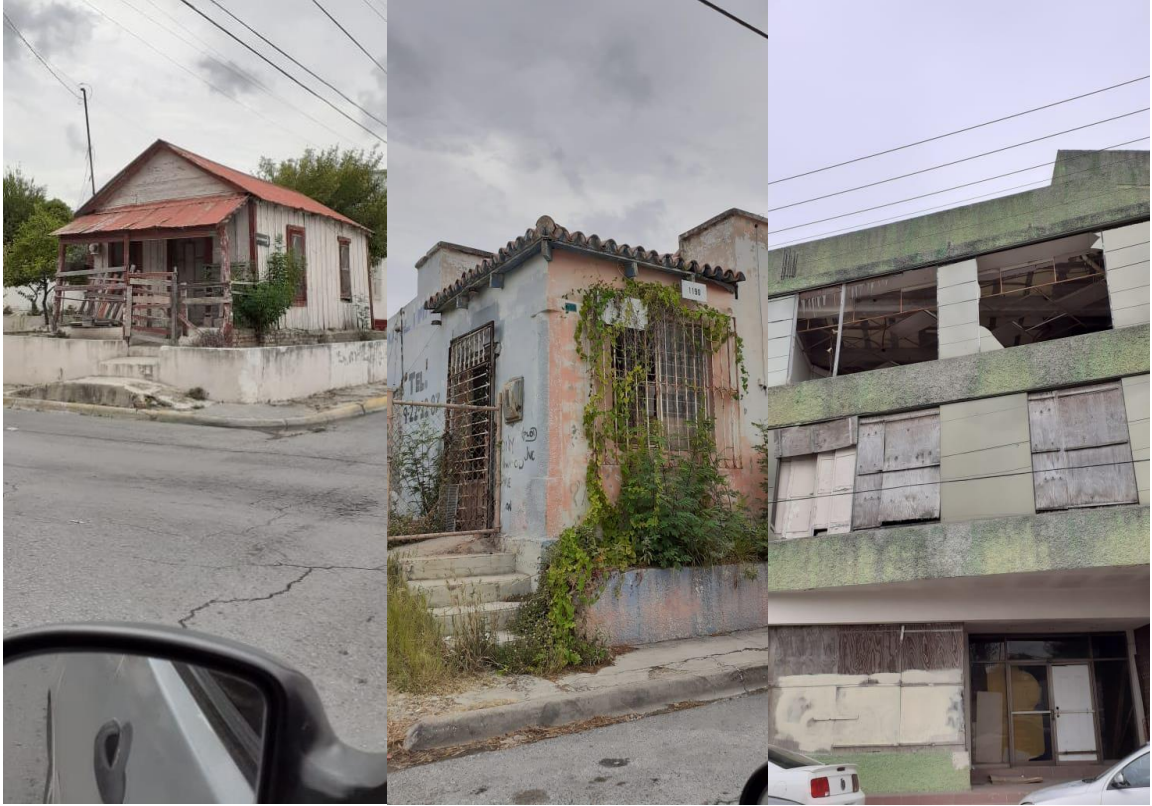
Figure B-2 Own Photographs. Abandoned Housing: Zona Centro, Reynosa, Tamaulipas, Mexico (2019).
