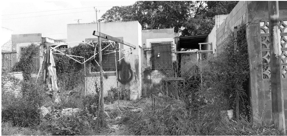
Figure B-13 Own Photographs. Abandoned Housing: Colonia Naranjitos, Reynosa, Tamaulipas, Mexico (2019).
