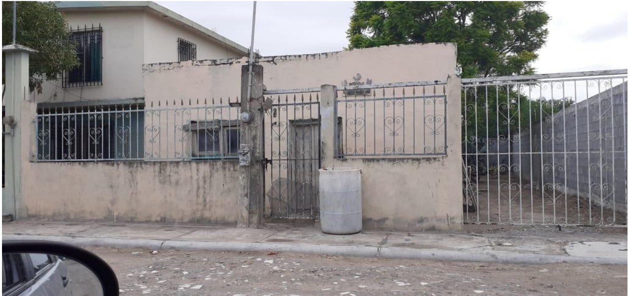
Figure B-16 Own Photographs. Abandoned Housing: Colonia Roma, Reynosa, Tamaulipas, Mexico (2019).
