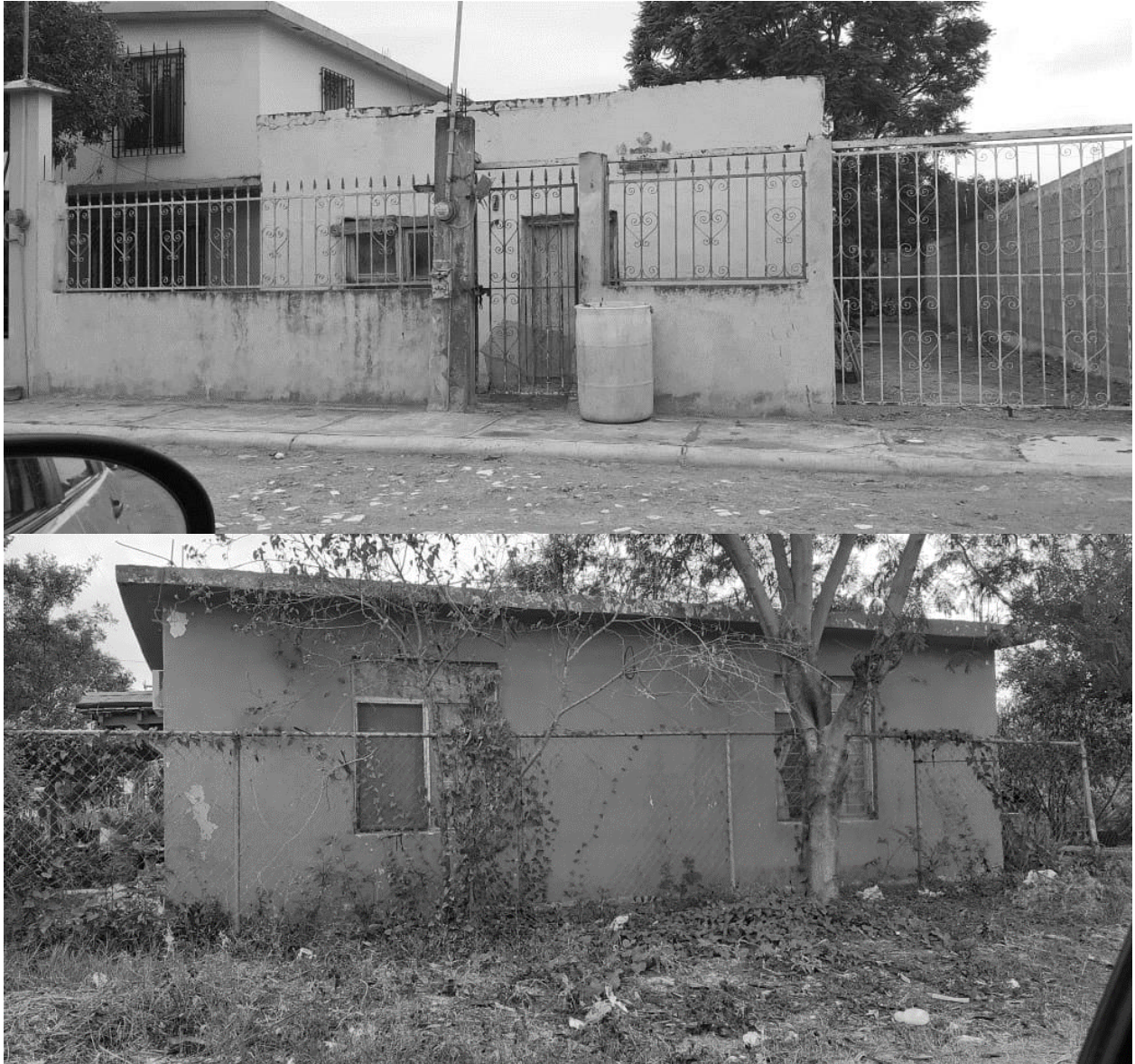
Figure B-8 Own Photographs. Abandoned Housing: Colonia Mexico, Reynosa, Tamaulipas, Mexico (2019).
