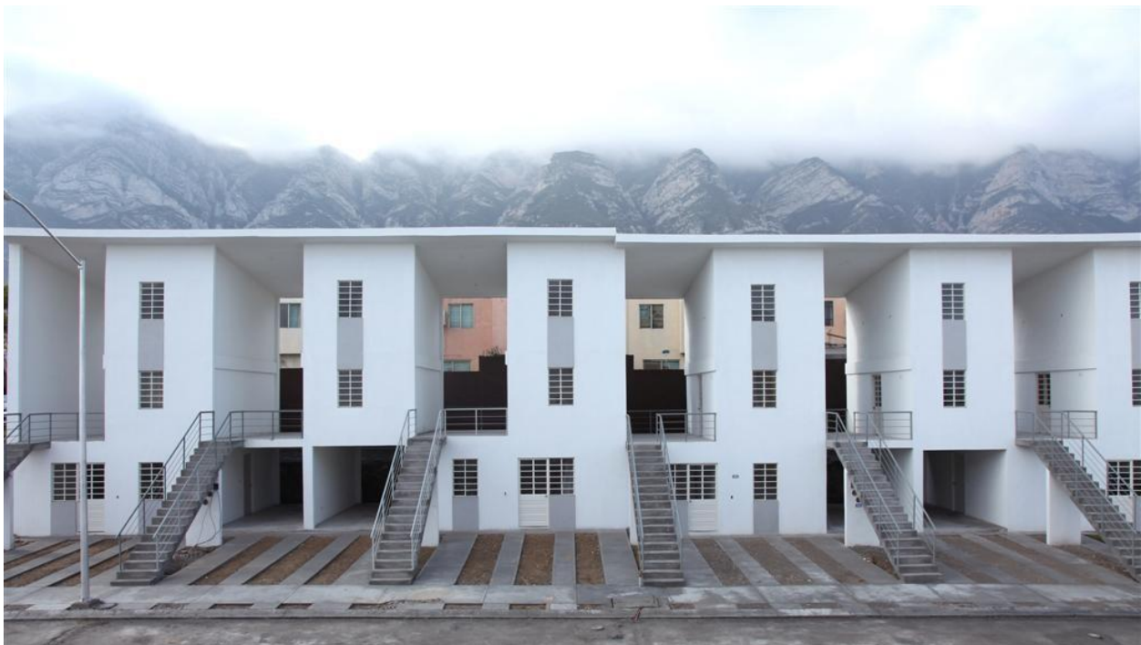
Figure 5.5 Elemental- Monterrey (facade) by Alejandro Aravena. Source: Reprinted from the website ArchDaily "Monterrey Housing / ELEMENTAL, 2010.
