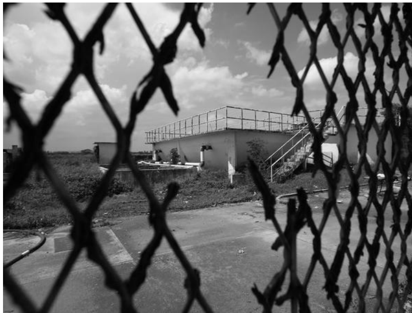
Figure 2.10 Not working water treatment plant at Colinas de Santa Fe in Veracruz, Mexico. Untreated sewage flows into a creek. Source: Reprinted from the LA Times article “Mexico’s Housing Debacle” by Richard Marosi, 2017. Photography by: Brian van der Brug Los Angeles Times, Marosi, 2017.
