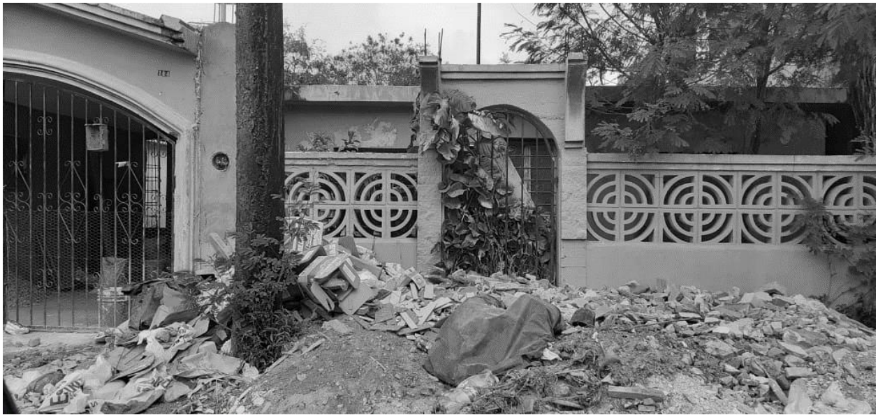
Figure B-15 Own Photographs. Abandoned Housing: Colonia Roma, Reynosa, Tamaulipas, Mexico (2019).
