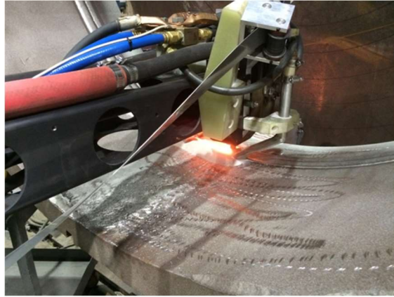
Figure 26 – Electro Slag Welding (ESW) of Strip on Carbon Steel Compressor Flange Face
