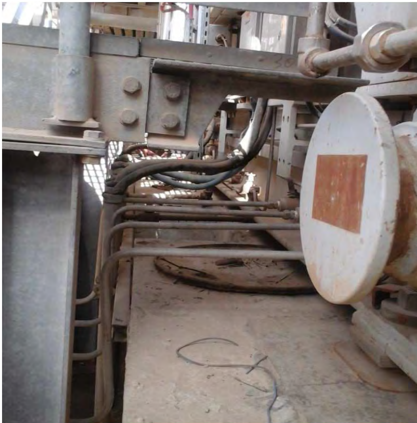
Before applying baseplate miniskirt
