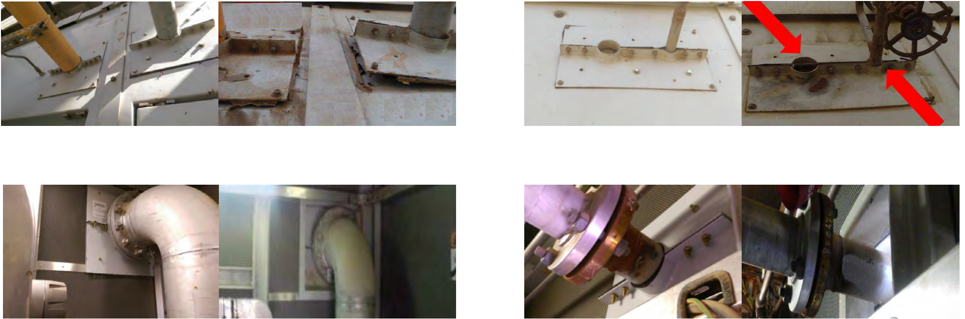
Gas turbine enclosure cross piping seal repairs and gasket replacement
