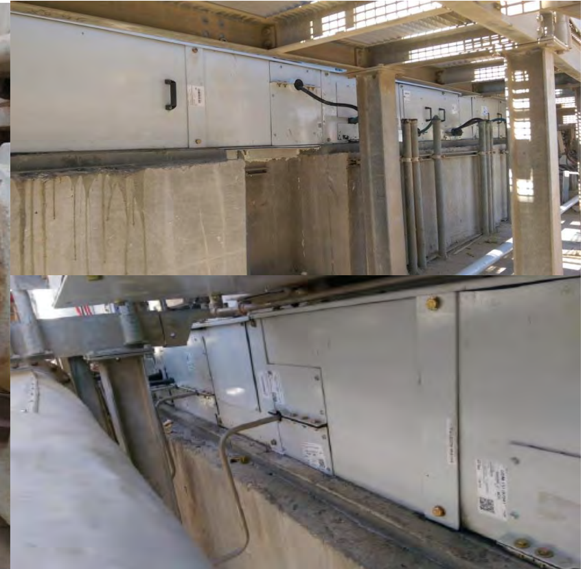
After applying baseplate miniskirt From back and front side of baseplate
