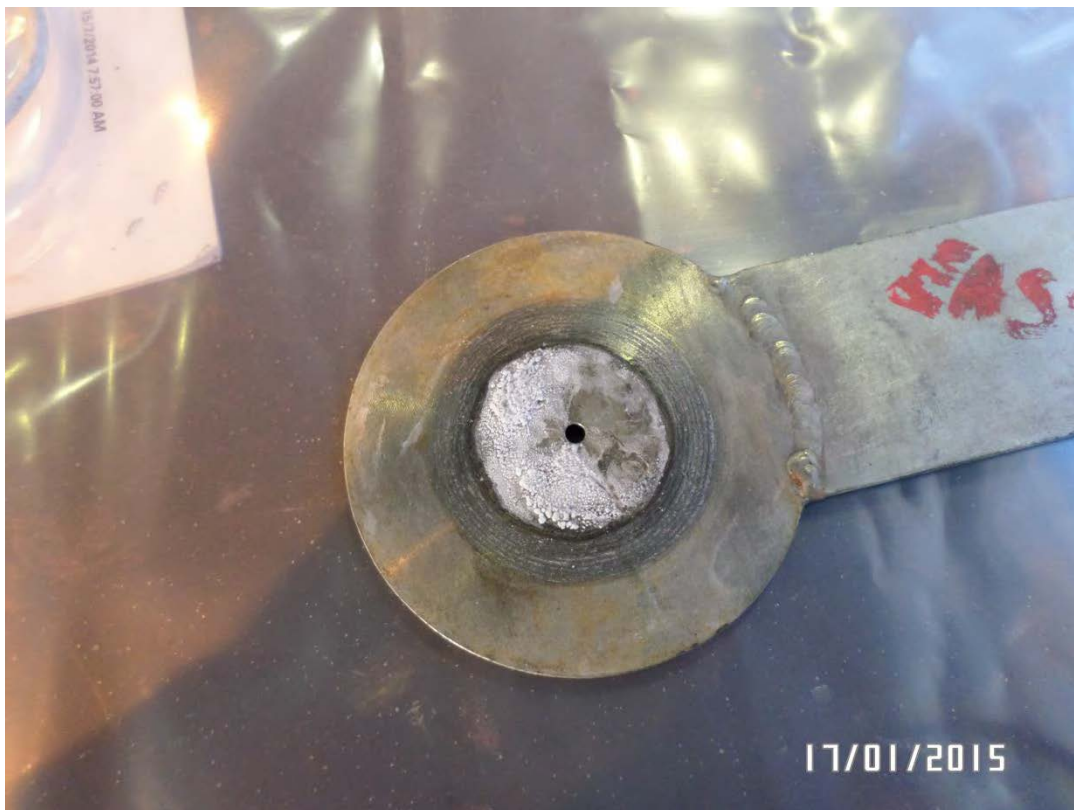
Chloride build up on the seal gas orifice plate
