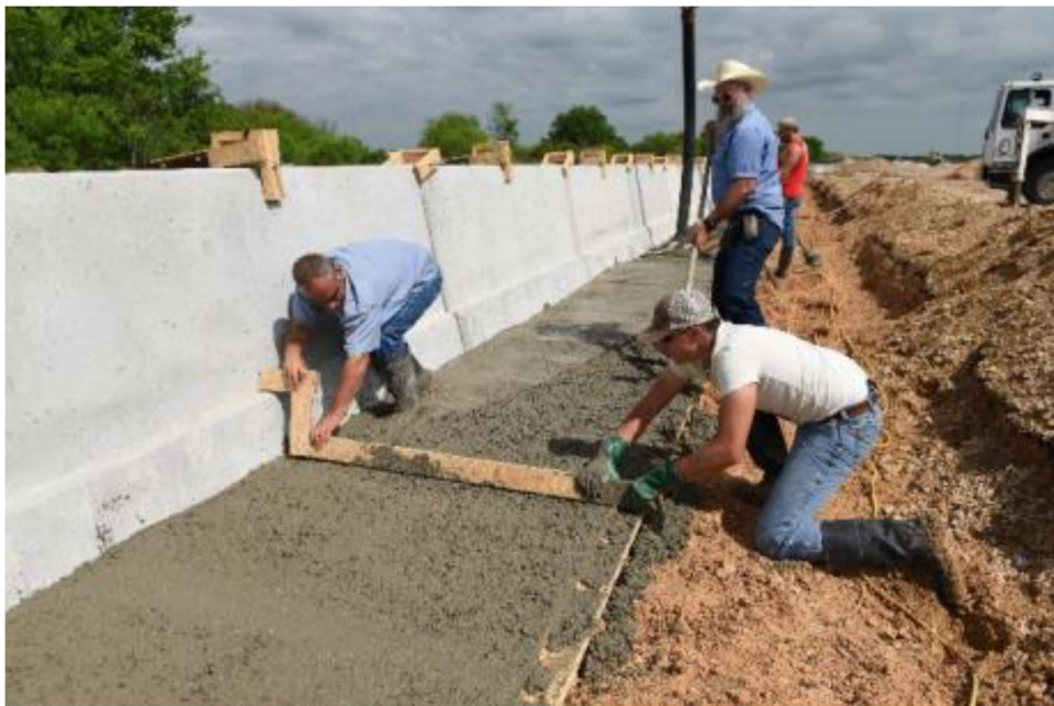
Figure 138 Casting of moment slab
