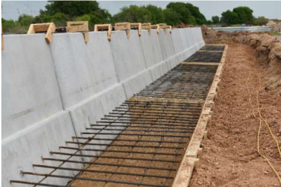
Figure 137 Moment-slab reinforcement
