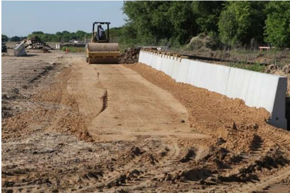
Figure 139 Compaction of fill in layers till finished ground level
