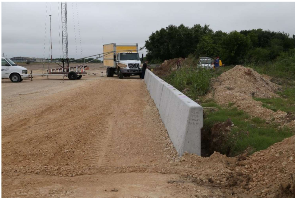
Figure 140 The finished TL-4 test installation
