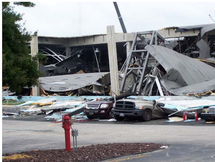
Figure 7: ConAgra Natural Gas Explosion and Ammonia Release 7
