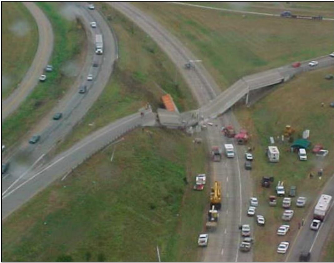
Figure 2. Impacted Bridge Pier by a Trailer-Truck in Dallas, Texas (TxDOT, 2001)
