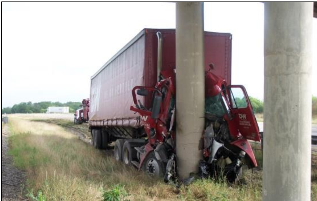
Figure 3. Bridge Pier Contains Heavy Vehicle in Dallas, Texas (TxDOT, 2007)
