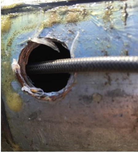
Figure 3-11: Drilled Borescope Inspection Hole
