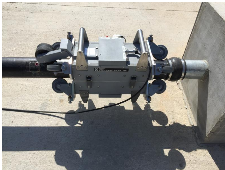
Figure 3-3: Installed LMA-450 Anchor Head
