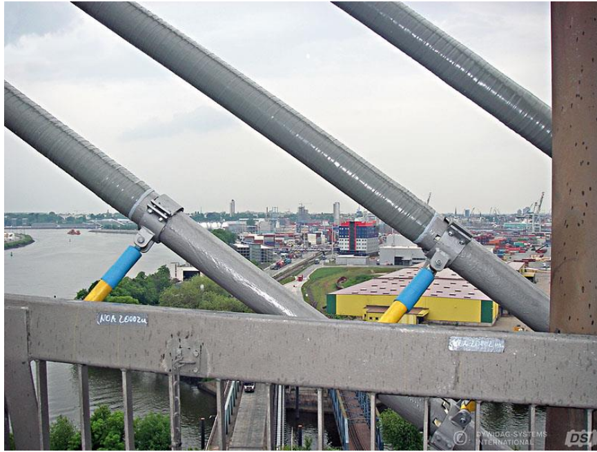
Figure 2-10: Repaired Corrosion Protection Coatings (DWIDAG-Systems International, 2014)
