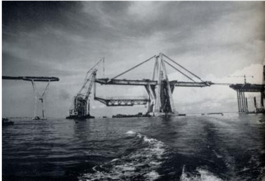
Figure 2-6: Construction operations during cable replacement (Pipinato, 2012)
