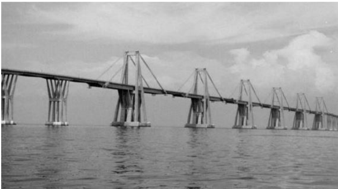
Figure 2-4: View of the Maracaibo Bridge (Pipinato, 2012)
