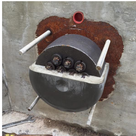
Figure 5-9: Partial Grouting of End Cap
