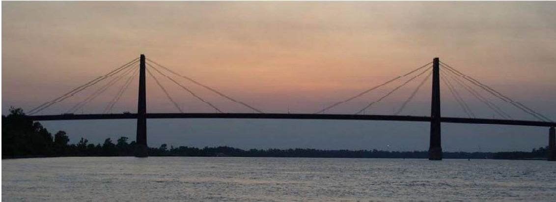
Figure 2-2: View of Luling Bridge (Mehrabi, 2009)
