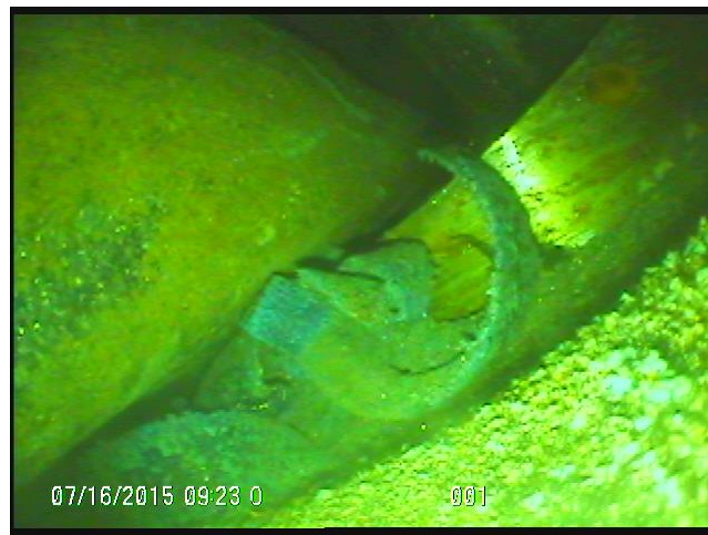
Figure B.6-12: Borescope Photo of Sheathing Stripping in Specimen 4 Grid I-J
