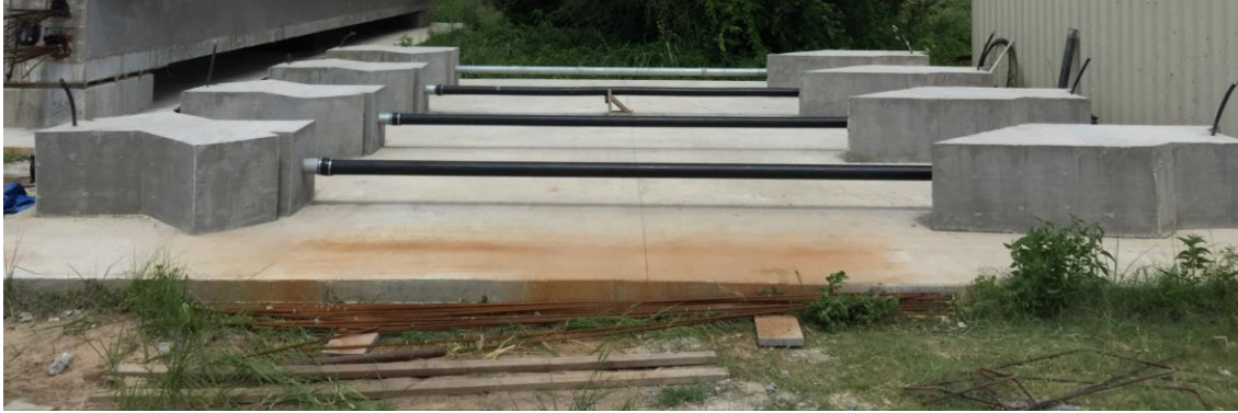
Figure 4-5: Completed Stay Cable Mock-Up Specimens
