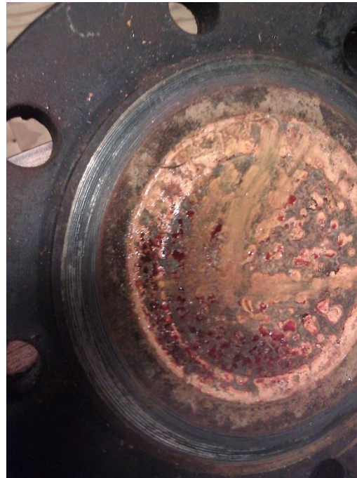
Figure 54: Flange damage and rust from shotgun pellets.
