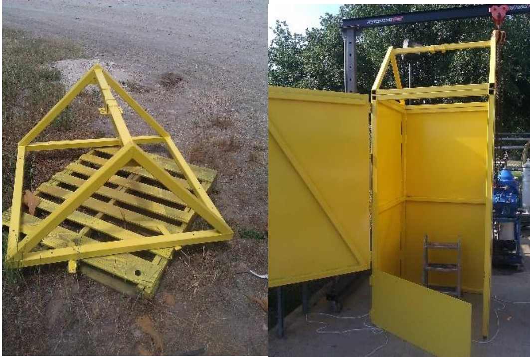
Figure 81: Bunker during installation.
