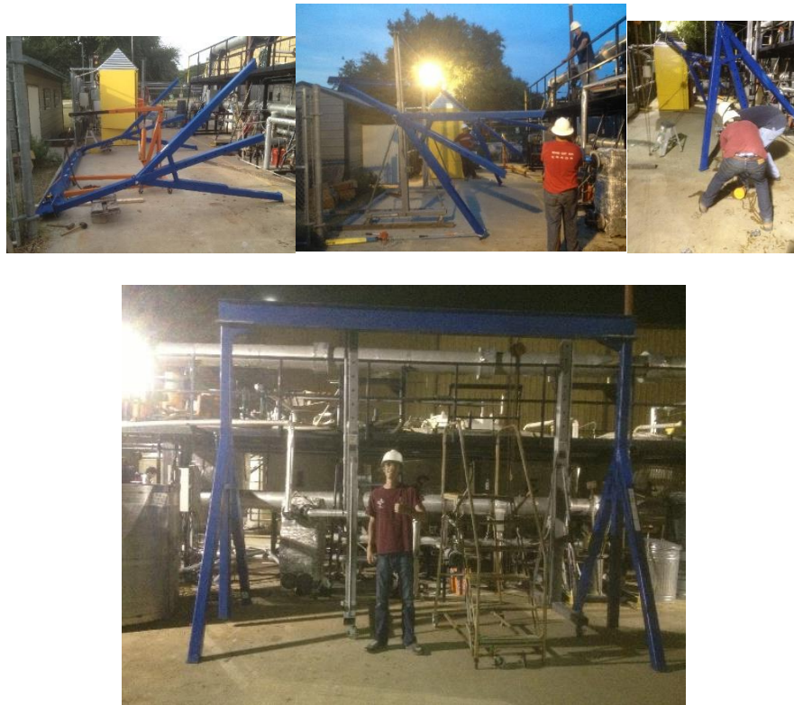
Figure 88: Erection of the 3-ton gantry crane (start to finish clockwise).
