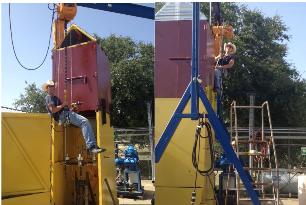
Figure 82: Installation of additional tower section on bunker.
