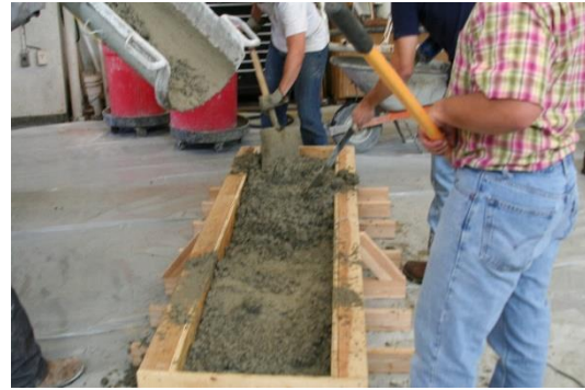
Figure 56. Casting From Truck - S9020NOS00
