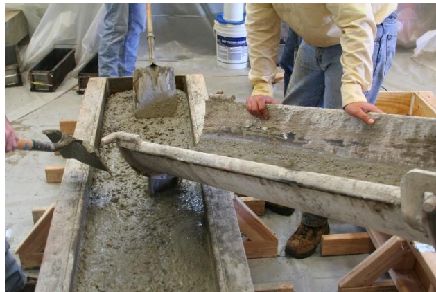
Figure 59. Placing Concrete Directly into Forms
