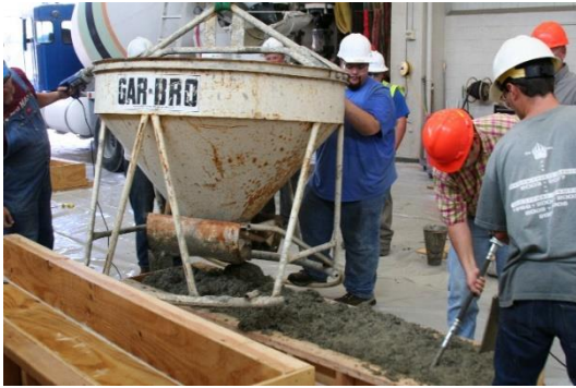
Figure 55. Casting from Hopper
