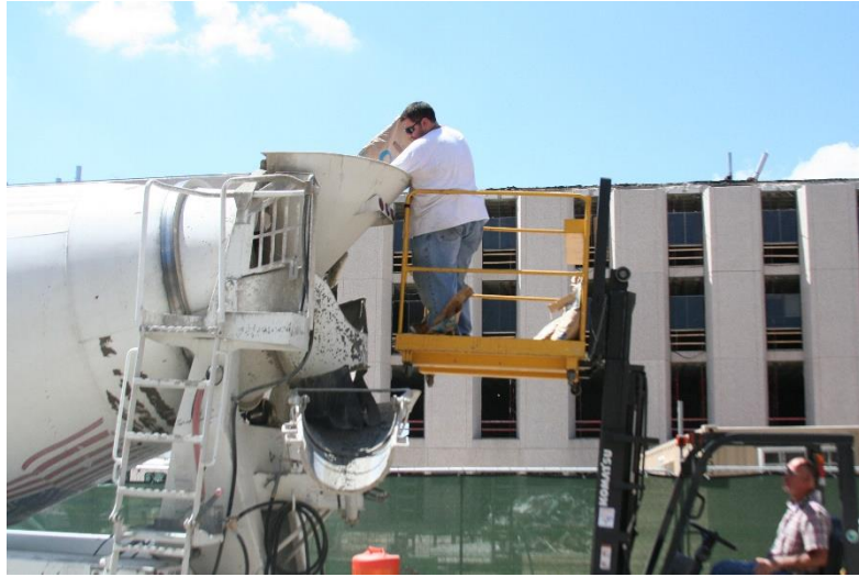
Figure 57. Adding Steel Fibers to Concrete Truck
