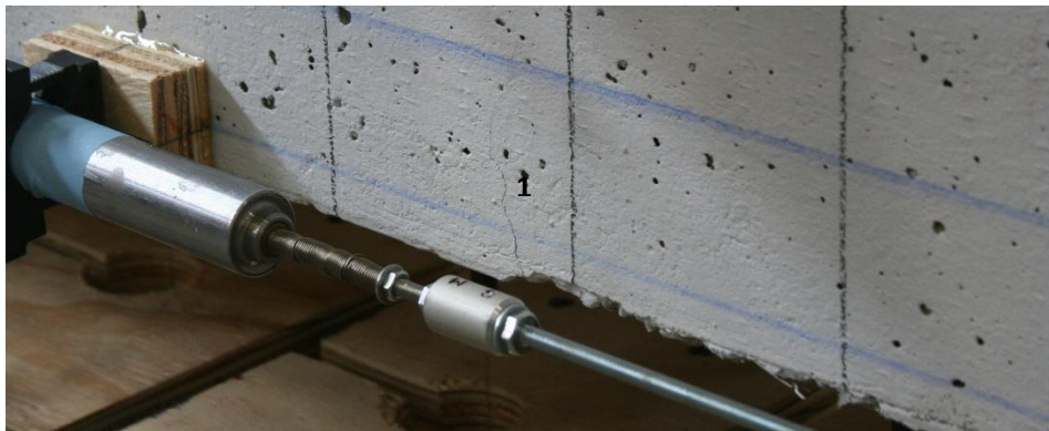
Figure 58. Damaged Corner of S7520NOS00 Where E1 Crack Formed
