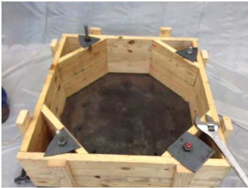
(a) Column Base Formwork Installation
