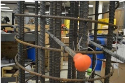
Figure 3.42. Temporary Dowel Formwork.
