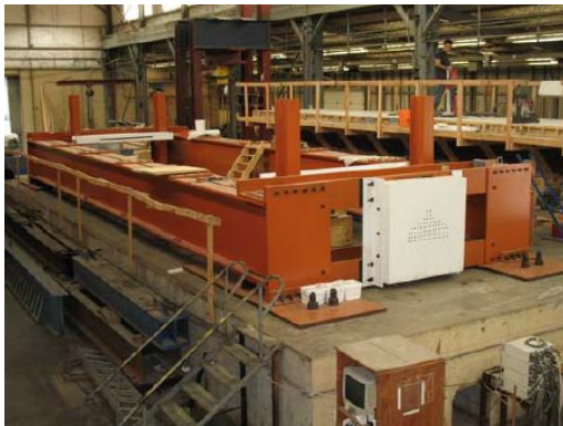
(a) Prestressing Bed
