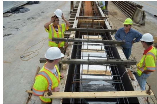
(b) Top Cover Plywood Cuts
