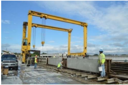
(a) Formwork Removal
