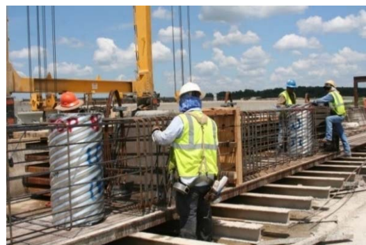
(b) Steel Corrugated Pipe
