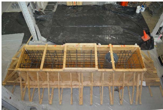
(c) Final Inspection
