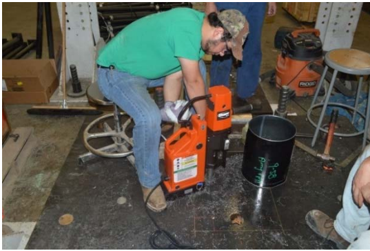
(a) Drilling 7/8-in holes
