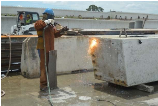
(a) Melting Strand Ends
