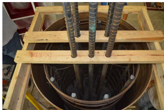
(b) Dowel Bars Supports
