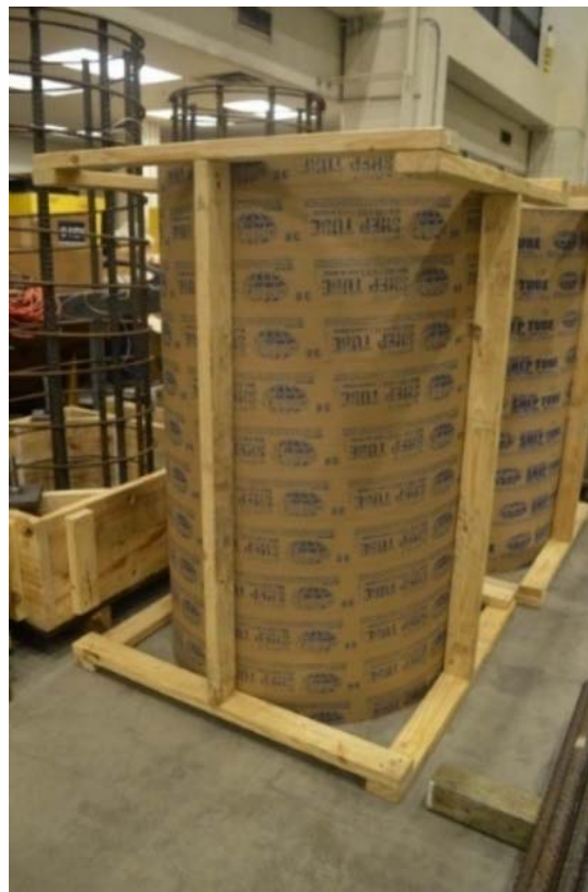
Figure 3.45. Column Sonotube Formwork.
