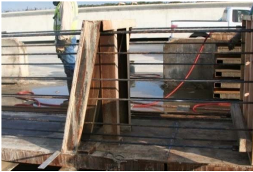
(a) Metal Formwork – Battered End
