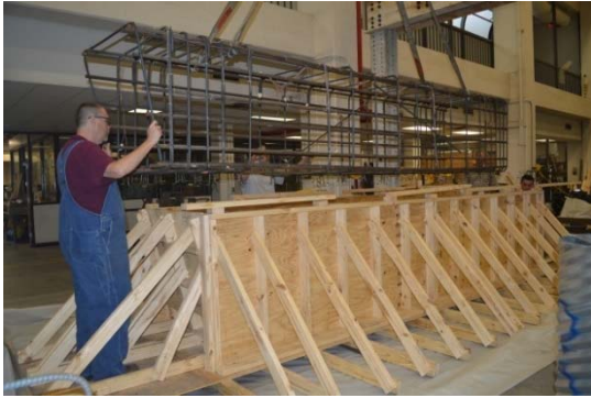
(a) Placing Steel Cage in Formwork
