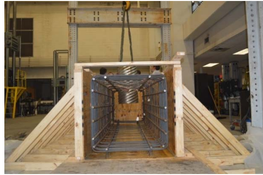
(b) Placing Corrugated Pipe
