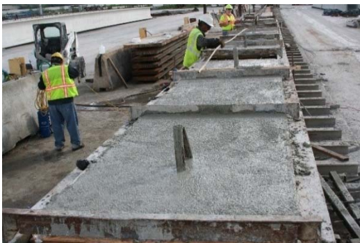
(a) Wood Trowel Finish
