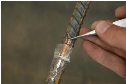
(c) Tape Strain Gage Installation
