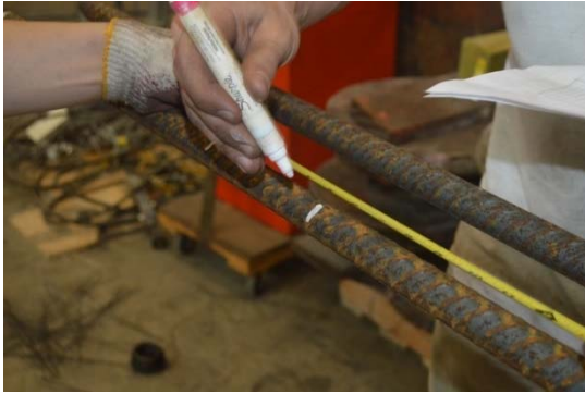
(a) Marking Location of S-bars
