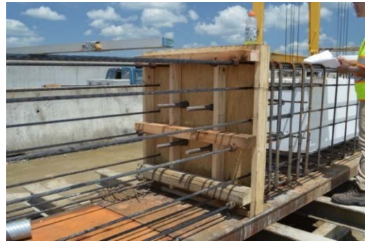
(b) Wood Formwork – Square End
