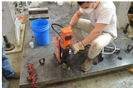
(b) Drilling 3-in Holes
