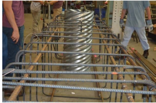
(b) Installed Bottom A-bars
