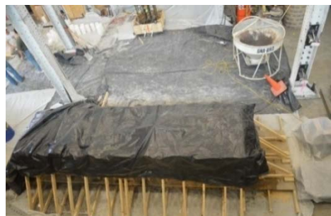
(h) Impermeable Curing Tarp
