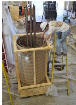
(a) Sonotube Installation
