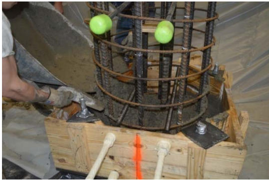
(a) Placement of Concrete with Wheel Barrels
