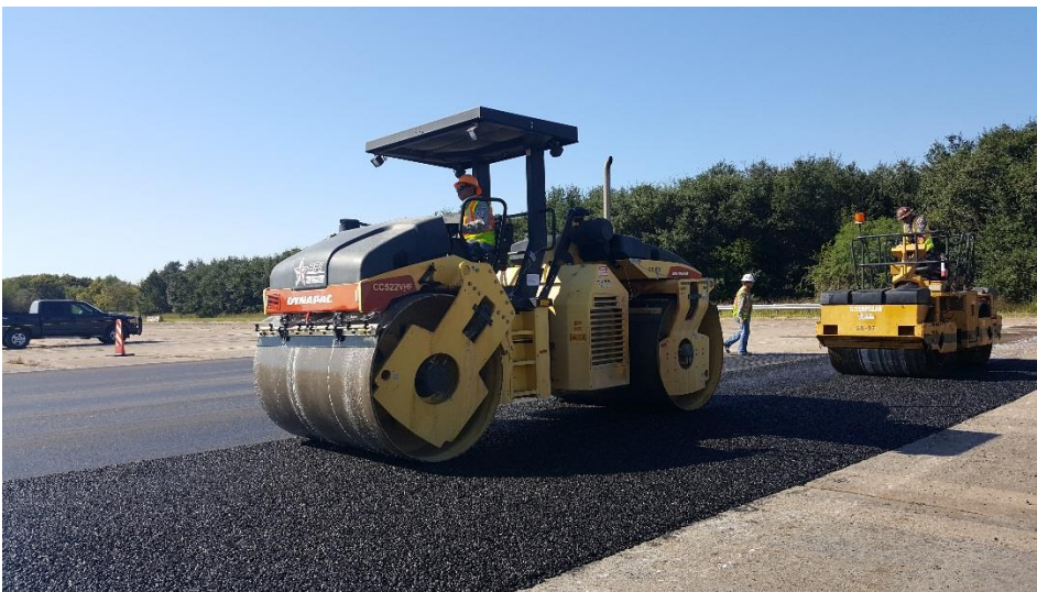
Figure G8. Compaction with two steel-wheeled roller in tandem.
