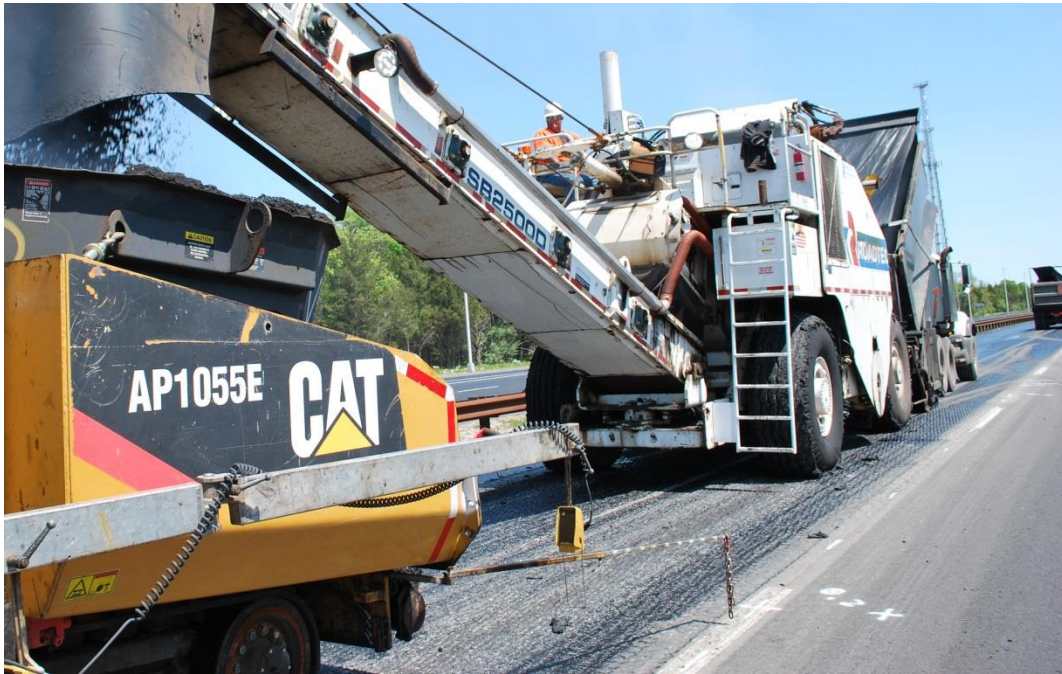
Figure F8. Picking of Tack by the Construction Equipment.
