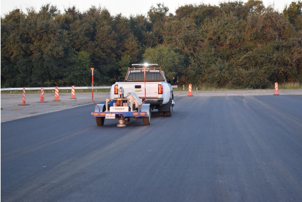
Figure G10. FWD Measurement at Test Pad.
