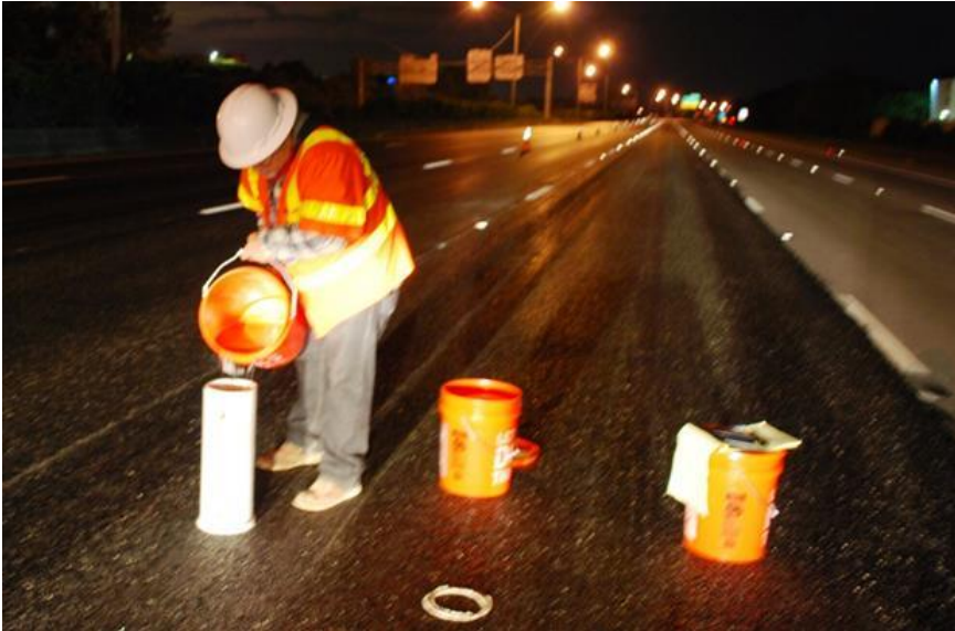
Figure D7. WFV test on right wheel path of lane R4.
