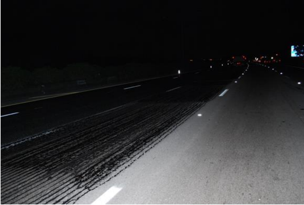
Figure D4. Tack coat application before placement of the OGFC mixture.
