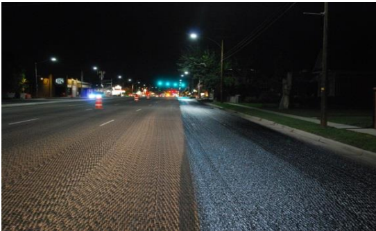
Figure 89. Milled surface.
