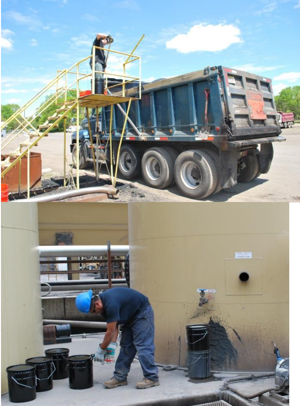
Figure F11. Collection of Plant Mix and Binder and Plant.
