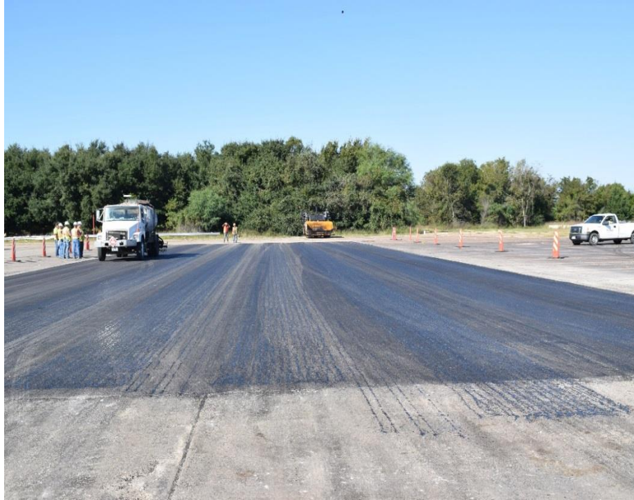
Figure G6. Tack Coat application prior to paving of OGFC layer.
