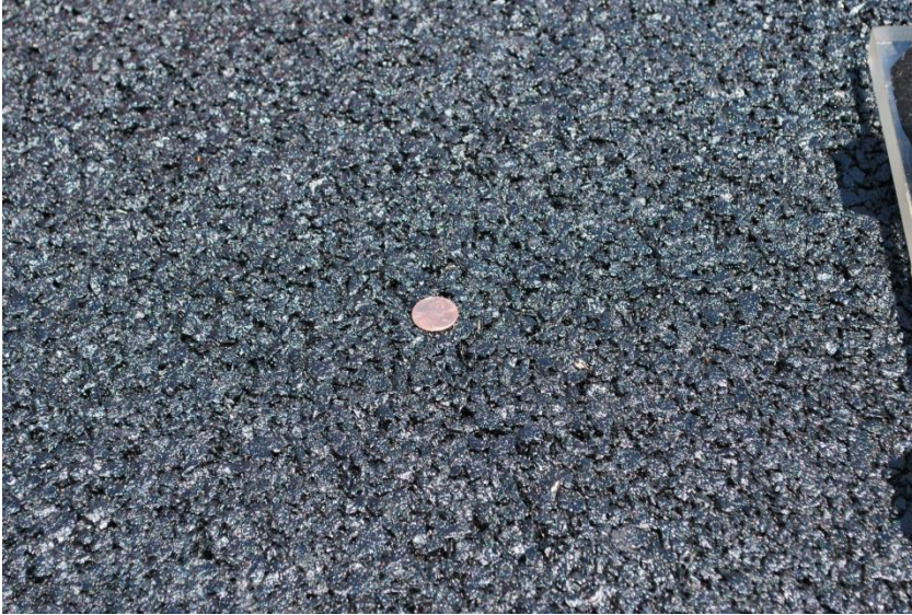
Figure F10. Close-up View of Freshly compacted Surface.
