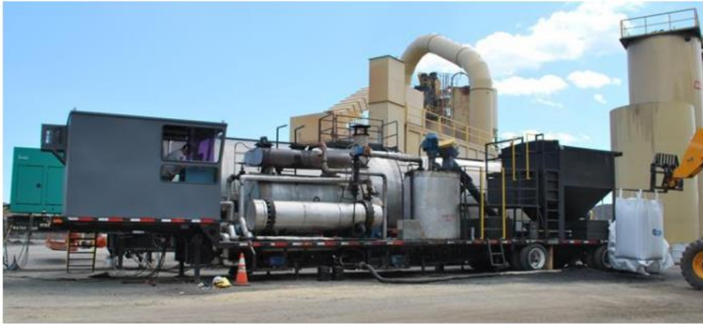
Figure 87. Portable crumb-rubber blending plant.
