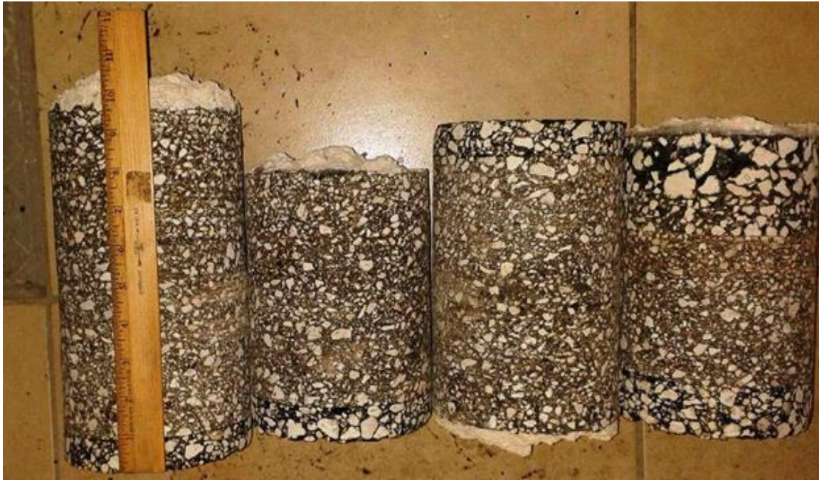
Figure D6. Field cores obtained after construction of the OGFC surface course on IH 95 in Florida.
