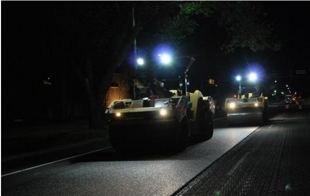
Figure E5. Paving of Friction Course on SR 71 in Utah.
